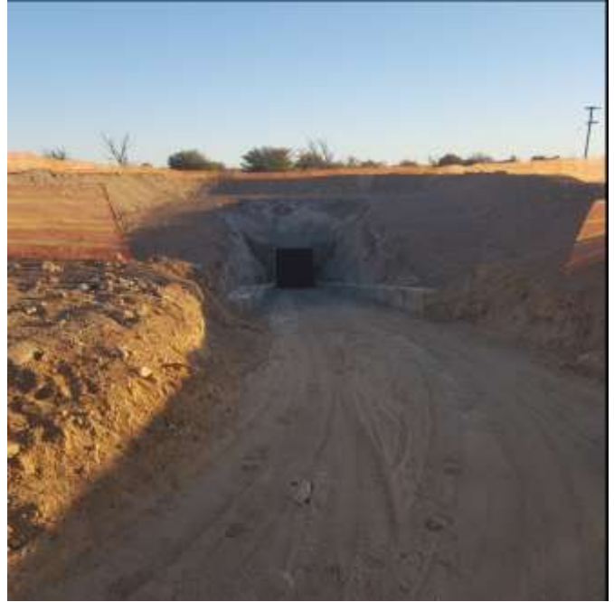
Decline Ramp Portal
