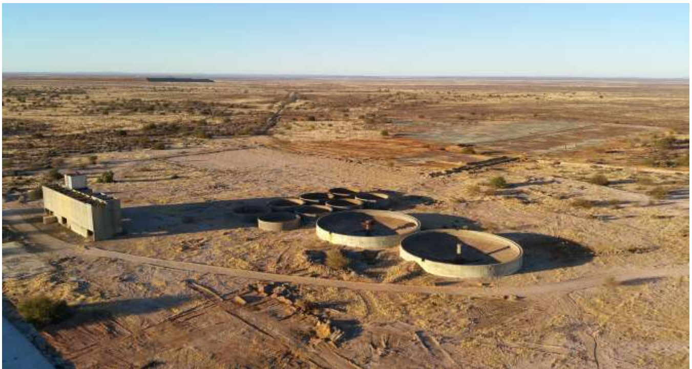
Crusher Bins, (left), Flotation Dams (middle foreground) and Concrete Drying Beds (right background)
