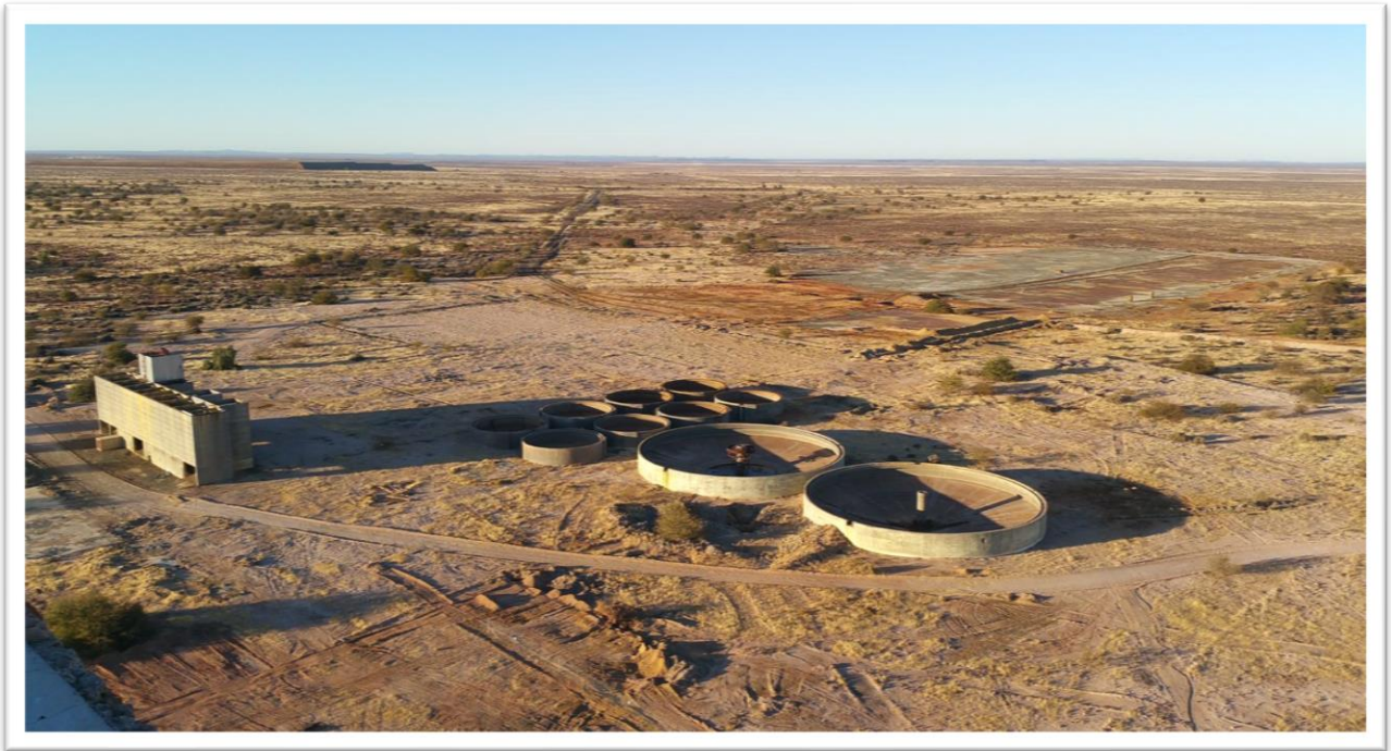
FIGURE 2: VIEW OF HISTORICAL ORE STOCKPILE BUNKER, CONCENTRATE THICKENERS AND CONCENTRATE DRYING BEDS FROM HUTCHINGS SHAFT
