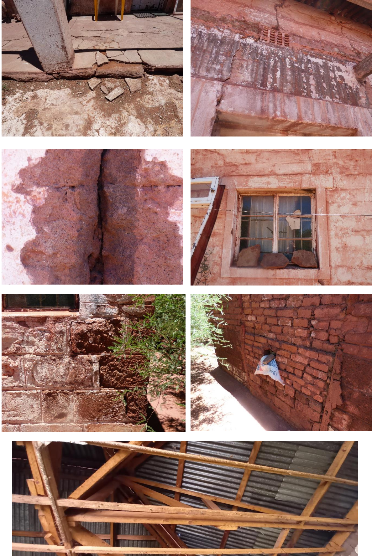
Figure 9 Details of structure's features
