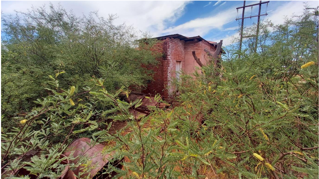
Figure 7 View of the southwest facade of the house
