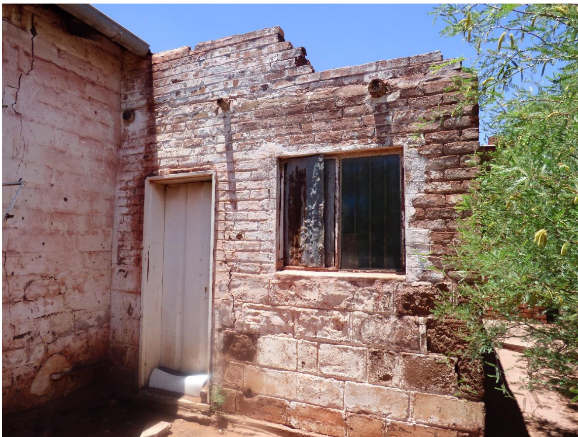
Figure 6 Southern facade addition
