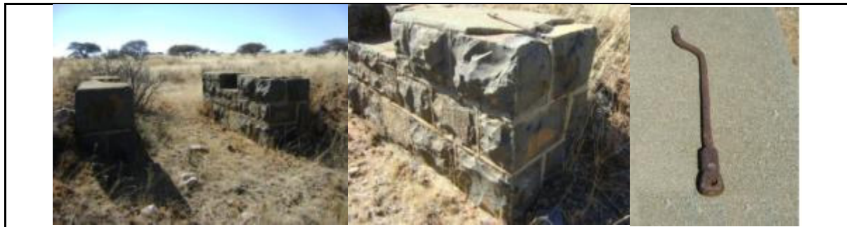
Figure 16: Along the road from the Ecco centre to the Olifantsfontein hotel there occurs a feature in the landscape. From other observations, it was a support structure for a water pipeline from the region where the steel reservoir is situated on the hill to the Wesselton mine. Culverts were built from dressed stone and period tools occur along the feature. (Photos S.M. Miller 2017.)
