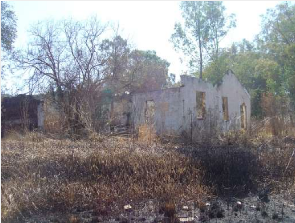
Figure 37 – Structure at MHC008 as documented in 2006.
