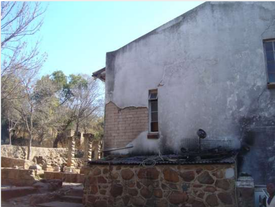
Figure 30 – Condition of the main house, circa 2006
