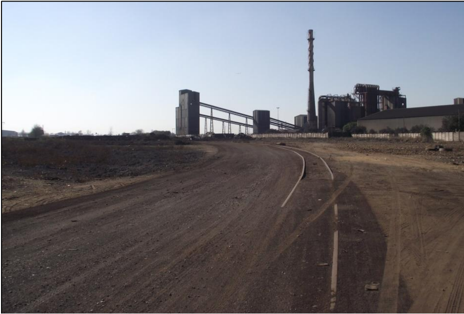
Figure 2 – Co-gen plant site, view from western boundary to south-east
