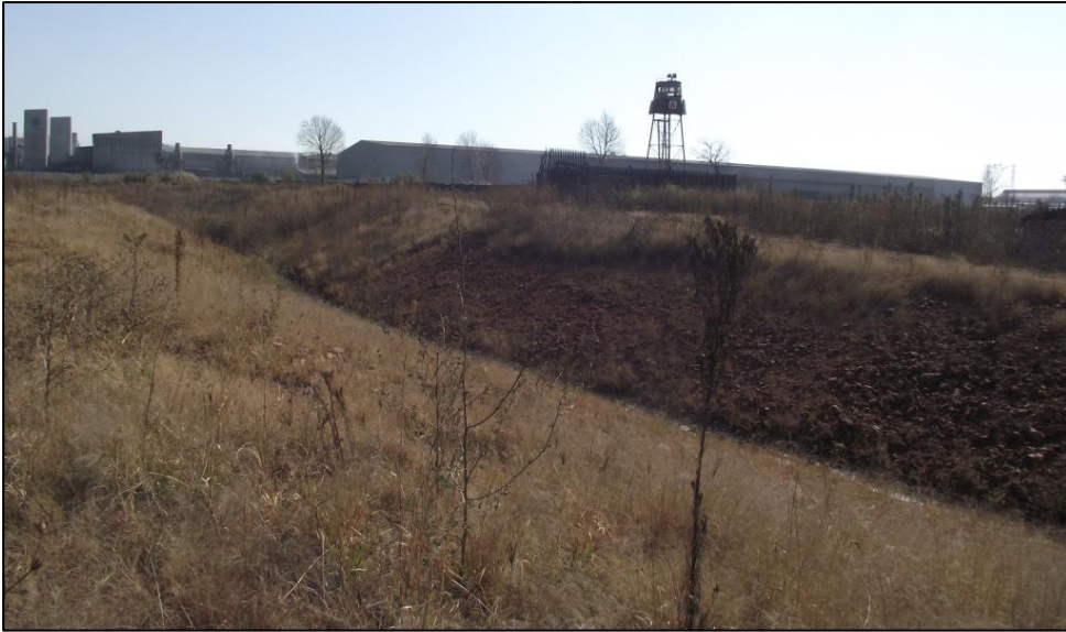
Figure 5 – Ash disposal site, showing drainage ditch in eastern section
