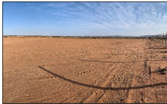
Figure 11: General view of PV plant area, looking east
