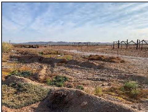
Figure 10: View of the PV plant area from the south-east
