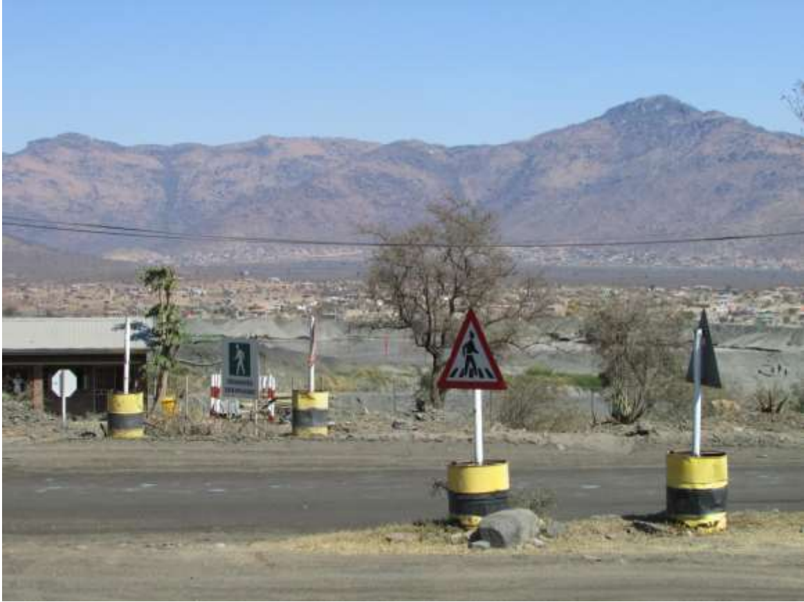
Figure 10: View of area close to existing Plant and WRD expansion area.
