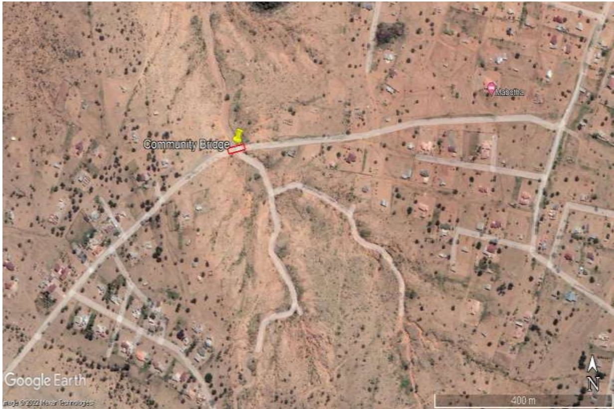
Figure 3: Another view of the location and footprint of the proposed bridge (Google Earth 2022).
