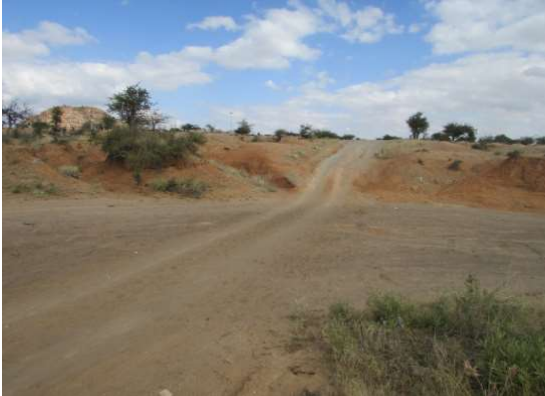
Figure 7: A view of the crossing where the Bokoni Community Bridge construction is proposed.
