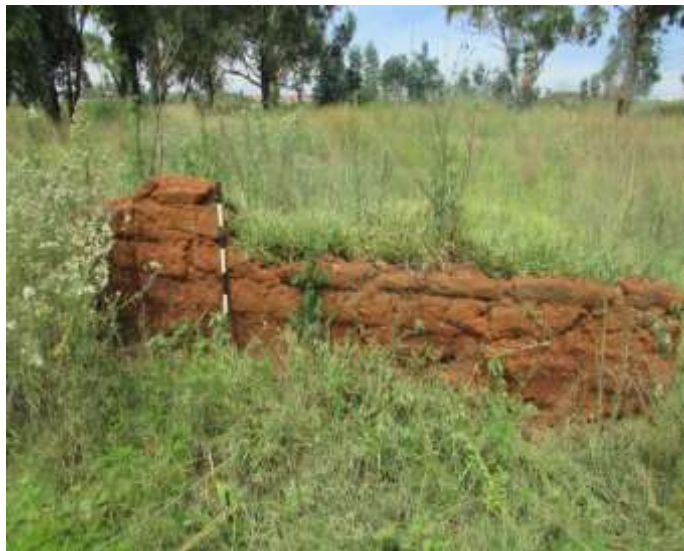
Fig.24: Remains of a clay-brick structure.
