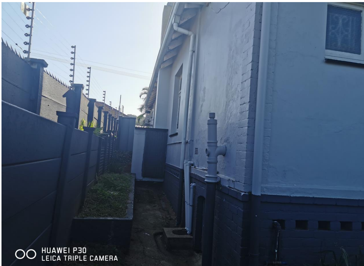
REAR VIEW OF OUTBUILDING
