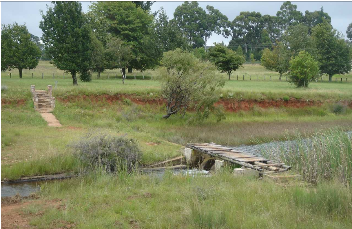
Existing Dam Wall
