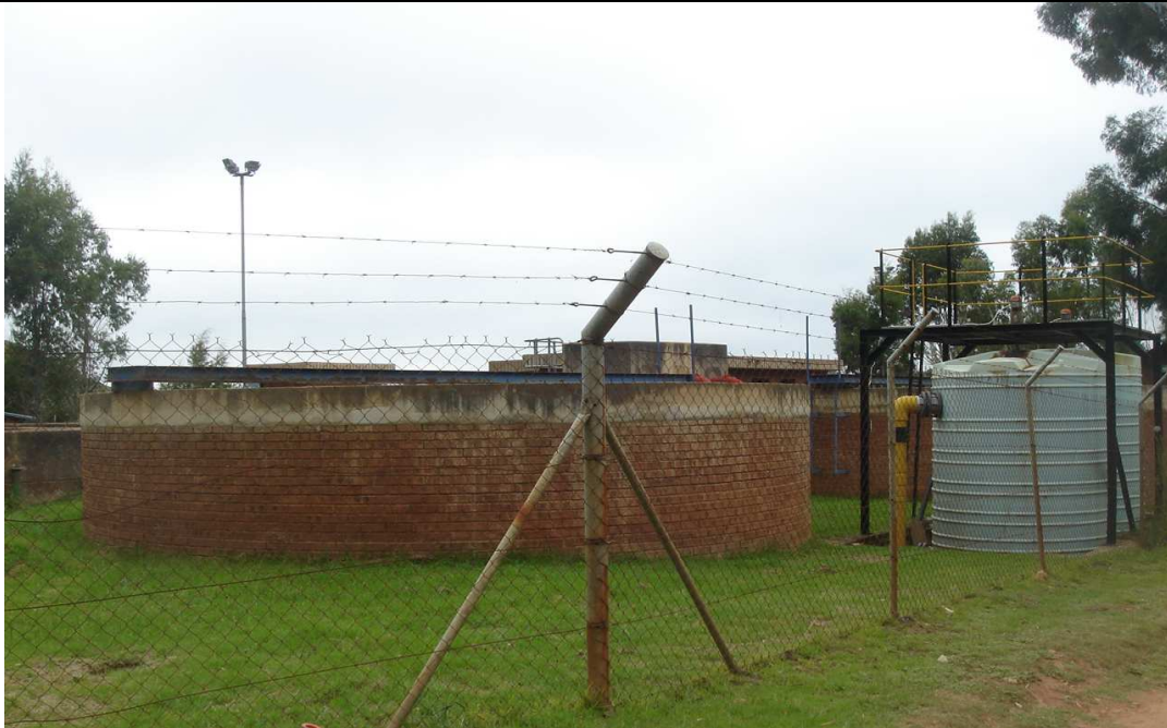
Dullstroom Water Treatment Works
