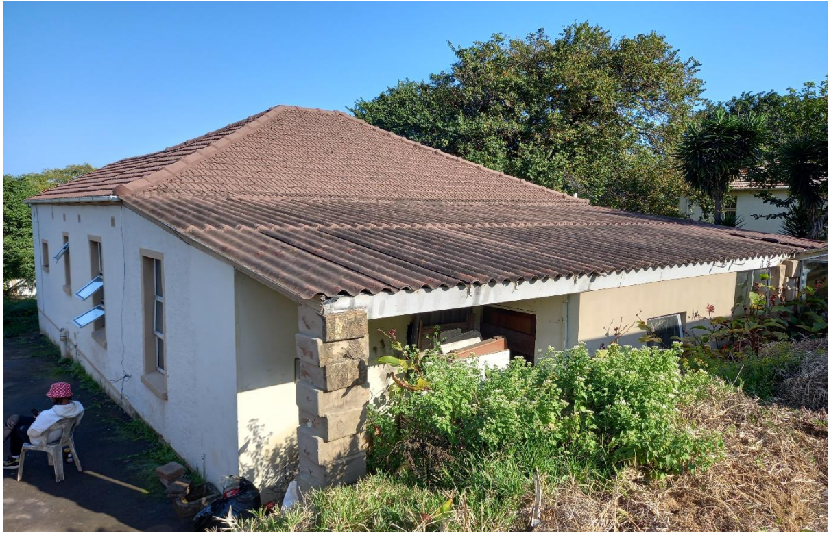
REAR OF BUILDING NORTH EAST ELEVATION
