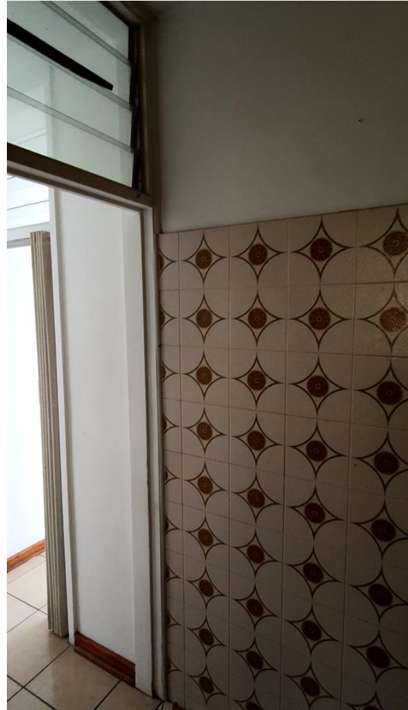
Figures 9 & 10. Image illustrates view of existing kitchen and its entrance. The kitchen shall be removed and converted to a new bedroom with en-suite as shown on the plan. The existing cupboards have swelled up over time and the tiles have become too slipper. Renovations will therefore be required to ensure safety.
