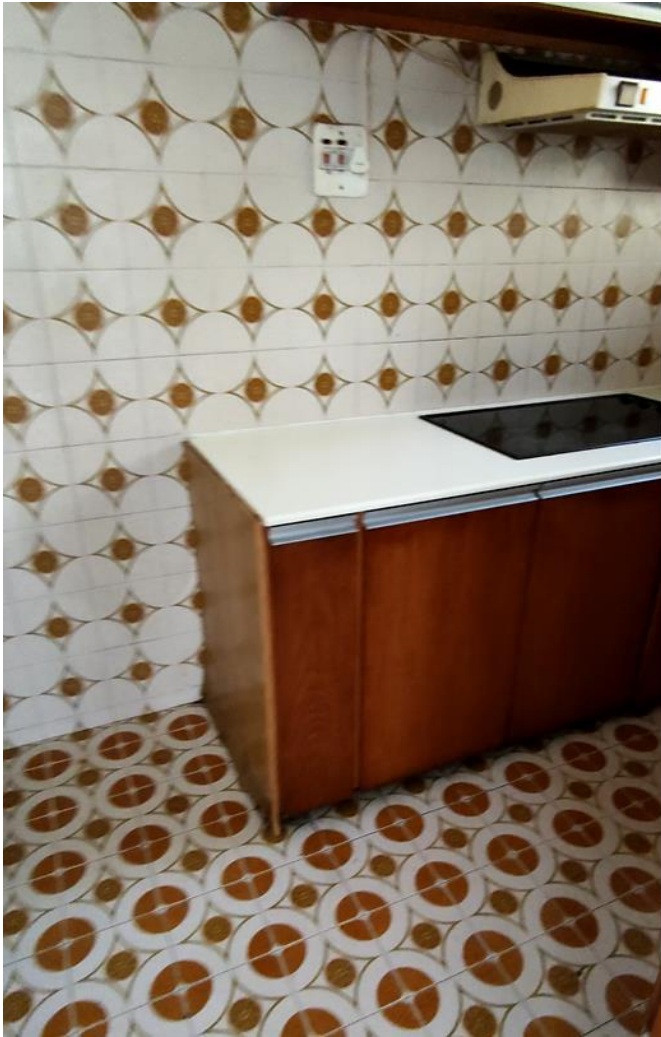
Figures 9 & 10. Image illustrates view of existing kitchen and its entrance. The kitchen shall be removed and converted to a new bedroom with en-suite as shown on the plan. The existing cupboards have swelled up over time and the tiles have become too slipper. Renovations will therefore be required to ensure safety.
