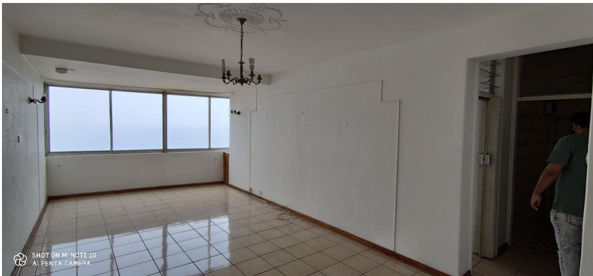
Figure 2. Image illustrates the existing lounge/dining as well as the passage, entrance to the bedroom and the existing kitchen (which shall be converted to a new en-suite, per the plan)
