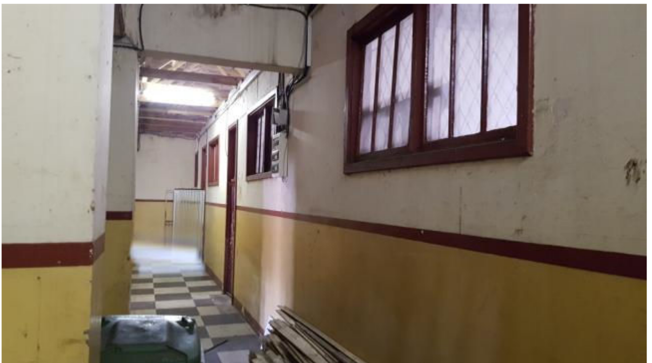
INTERIOR FIRST FLOOR PASSAGE
