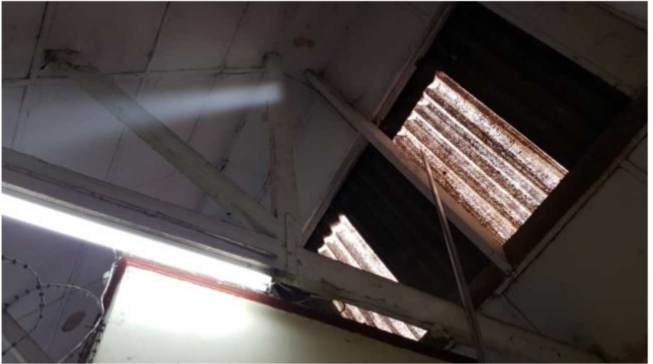
INTERIOR – FIRST FLOOR ROOF TRUSSES
