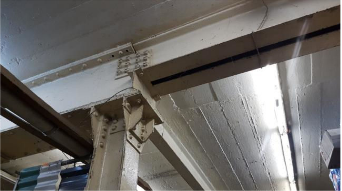
INTERIOR GROUND FLOOR
