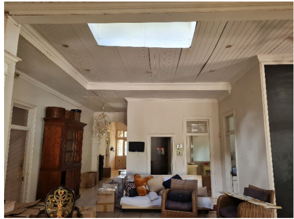
EXISTING LIVING ROOM
