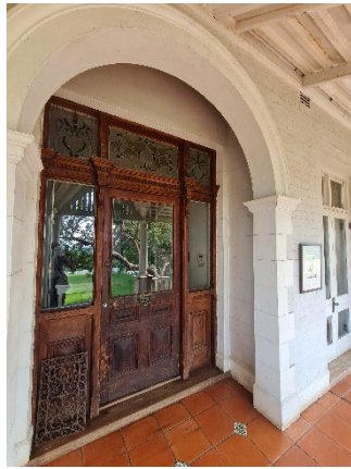
EXISTING ENTRANCE DOOR
