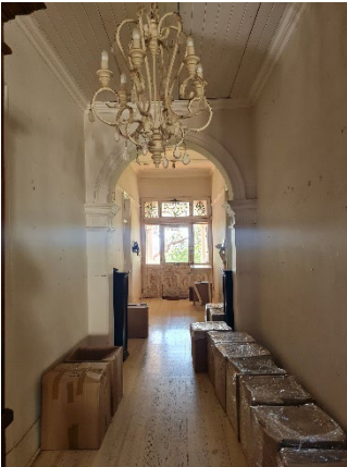
EXISTING HALLWAY LEADING TO FRONT DOOR
