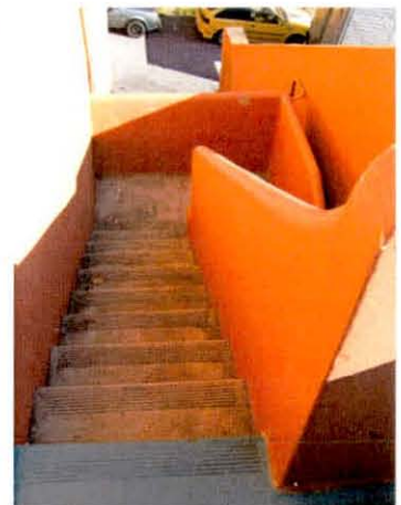
External escape stair.
