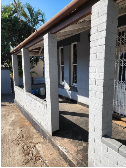
NORTH ELEVATION MAIN DWELLING SHOWING EXISTING VERANDAH .
