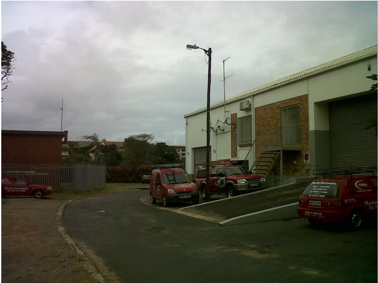
Southeast from pumpstation 3A
