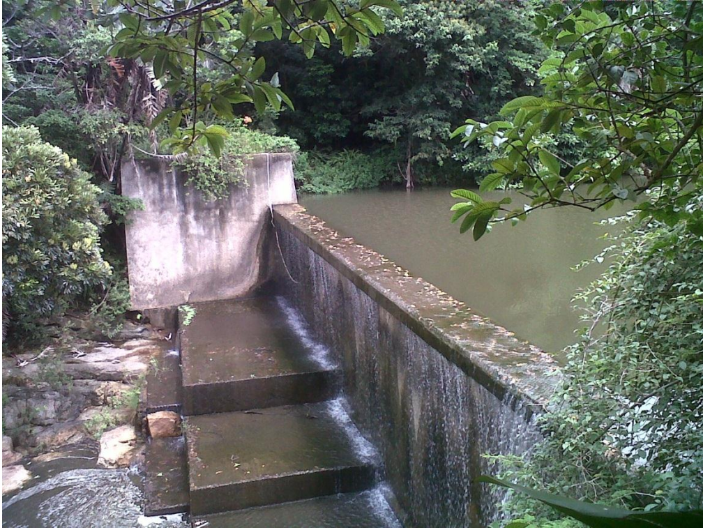
Pic showing weir at Inkongweni Stream
