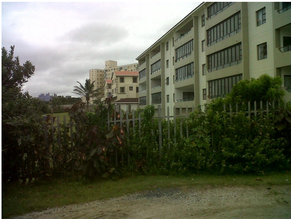
Holiday flats-reticulation to be rerouted away from private property
