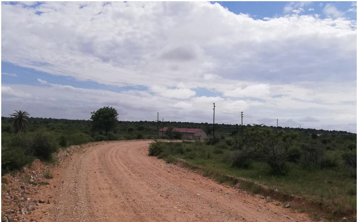
Photo 1: Shows the gravel road and existing poles and a house
