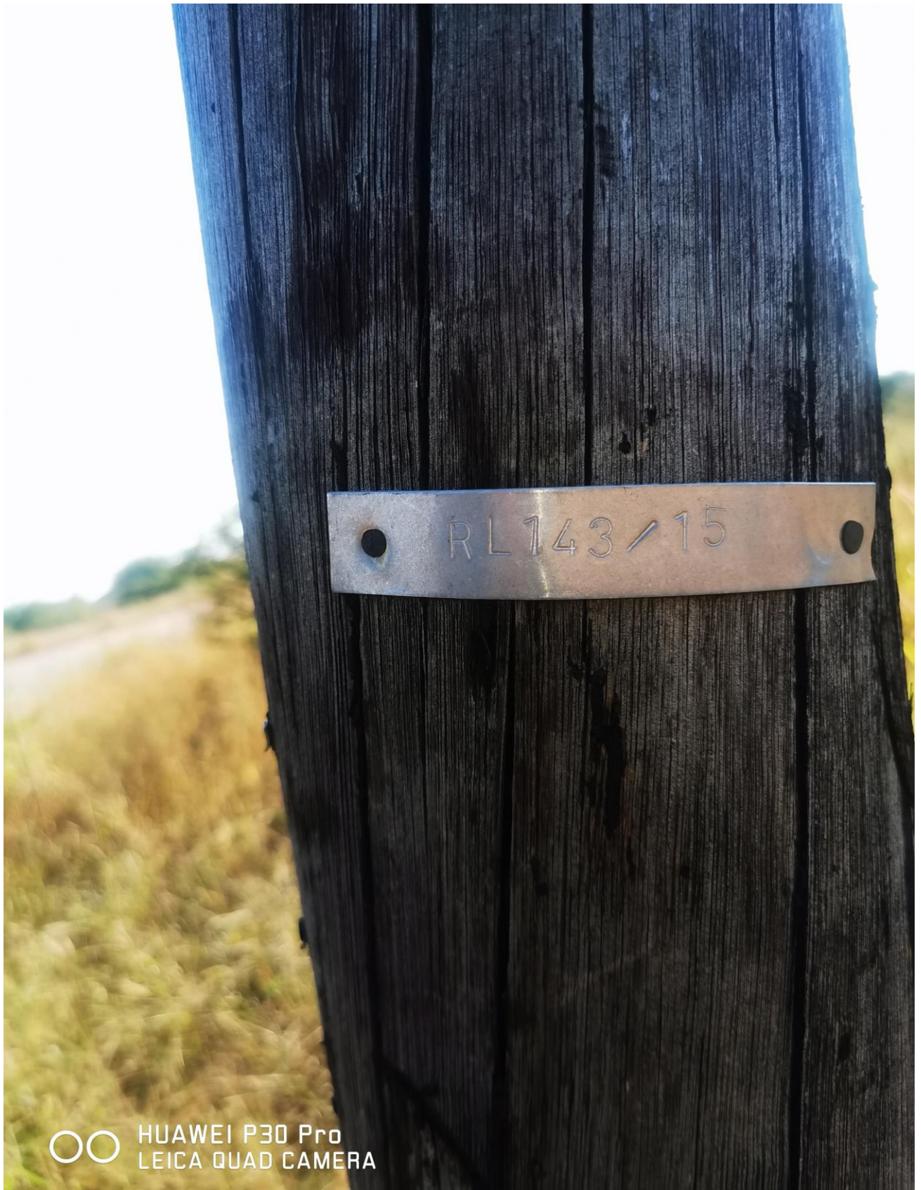
Figure 1: Existing line from the proposed project
