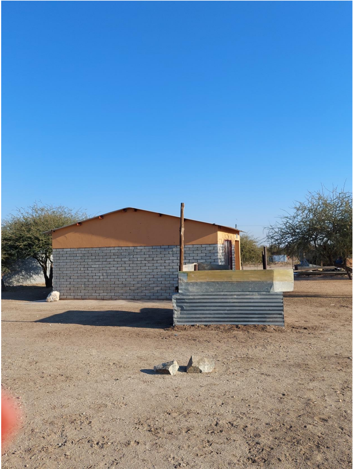
Figure 4: Picture showing one of the houses to be supplied with electricity
