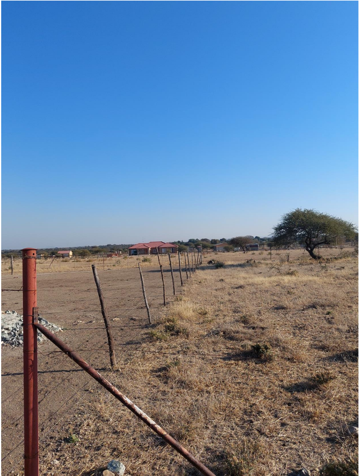
Figure 10: A picture showing where the lower voltage lines will be running behind the houses
