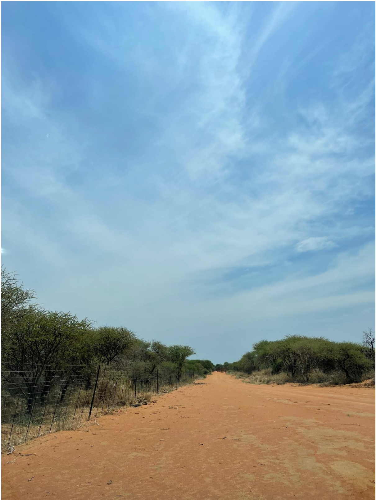
Figure 9: Picture showing existing road infrastructure
