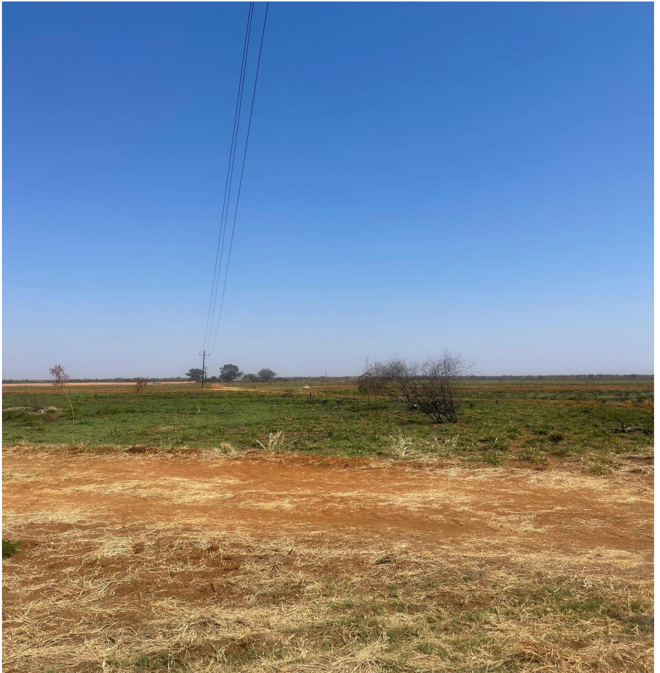
Figure 1: Picture showing the existing line in the area
