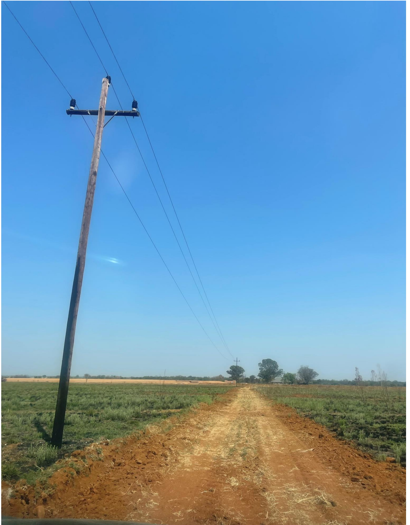
Figure 2: Another picture showing the existing line in the area
