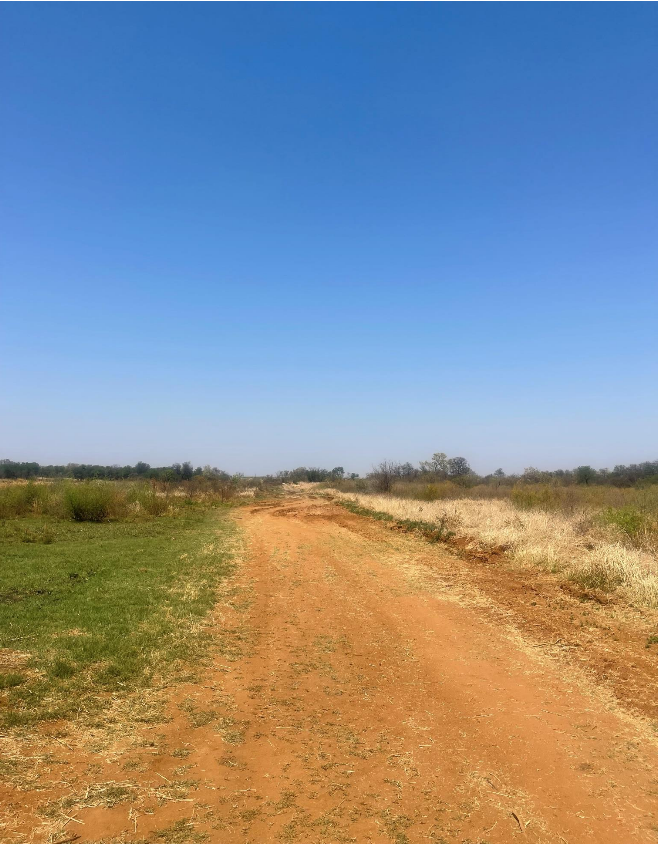
Figure 10: Picture showing the existing road infrastructure
