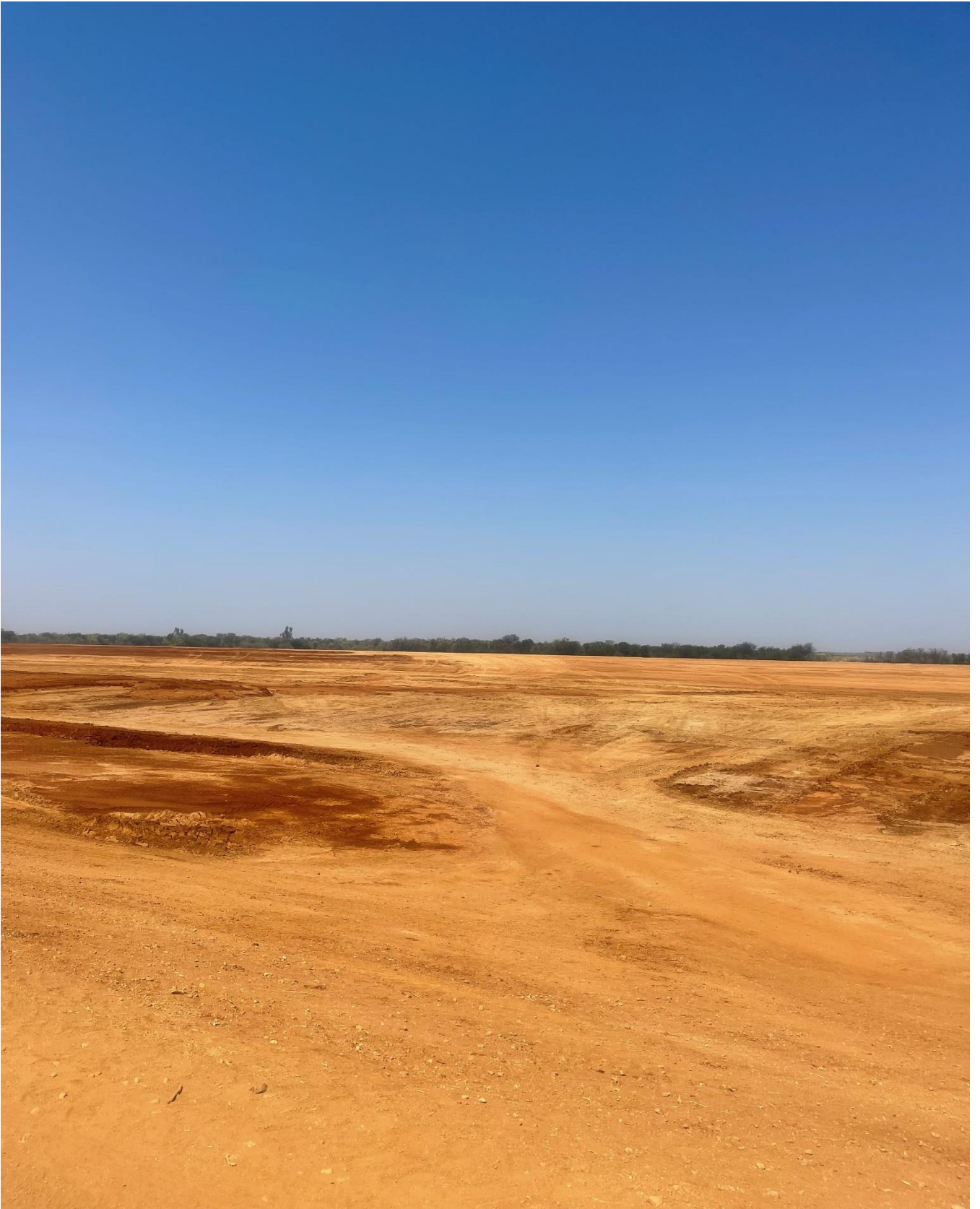
Figure 11: Picture showing the newly constructed dam
