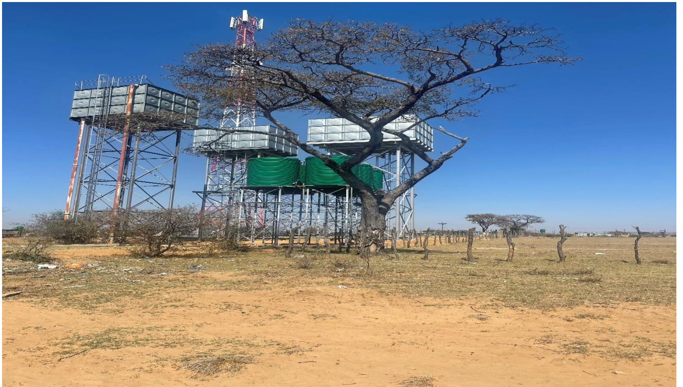
Figure 1: Picture showing the cell tower and water tank next to the existing T-Off line
