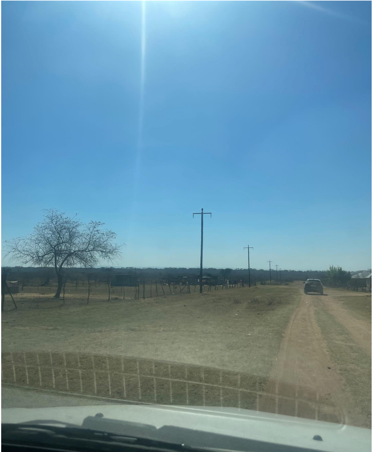
Figure 3: Picture showing the existing powerline in the project area
