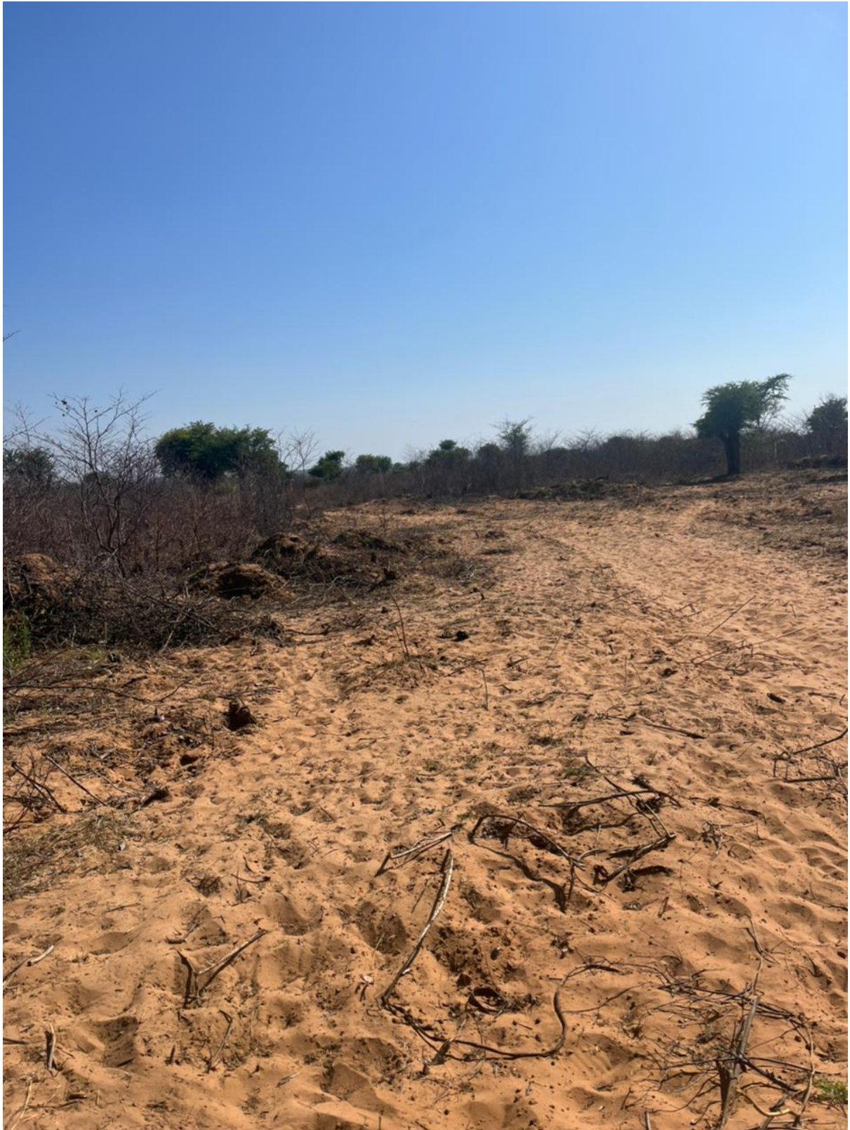
Figure 5: Picture showing pole position of the powerline
