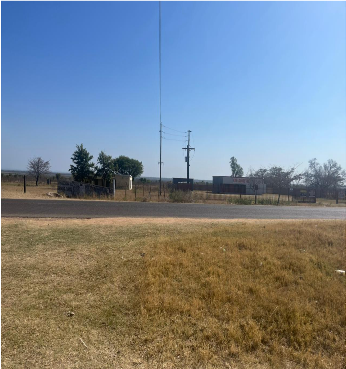
Figure 1: Picture showing existing electricity in the study area
