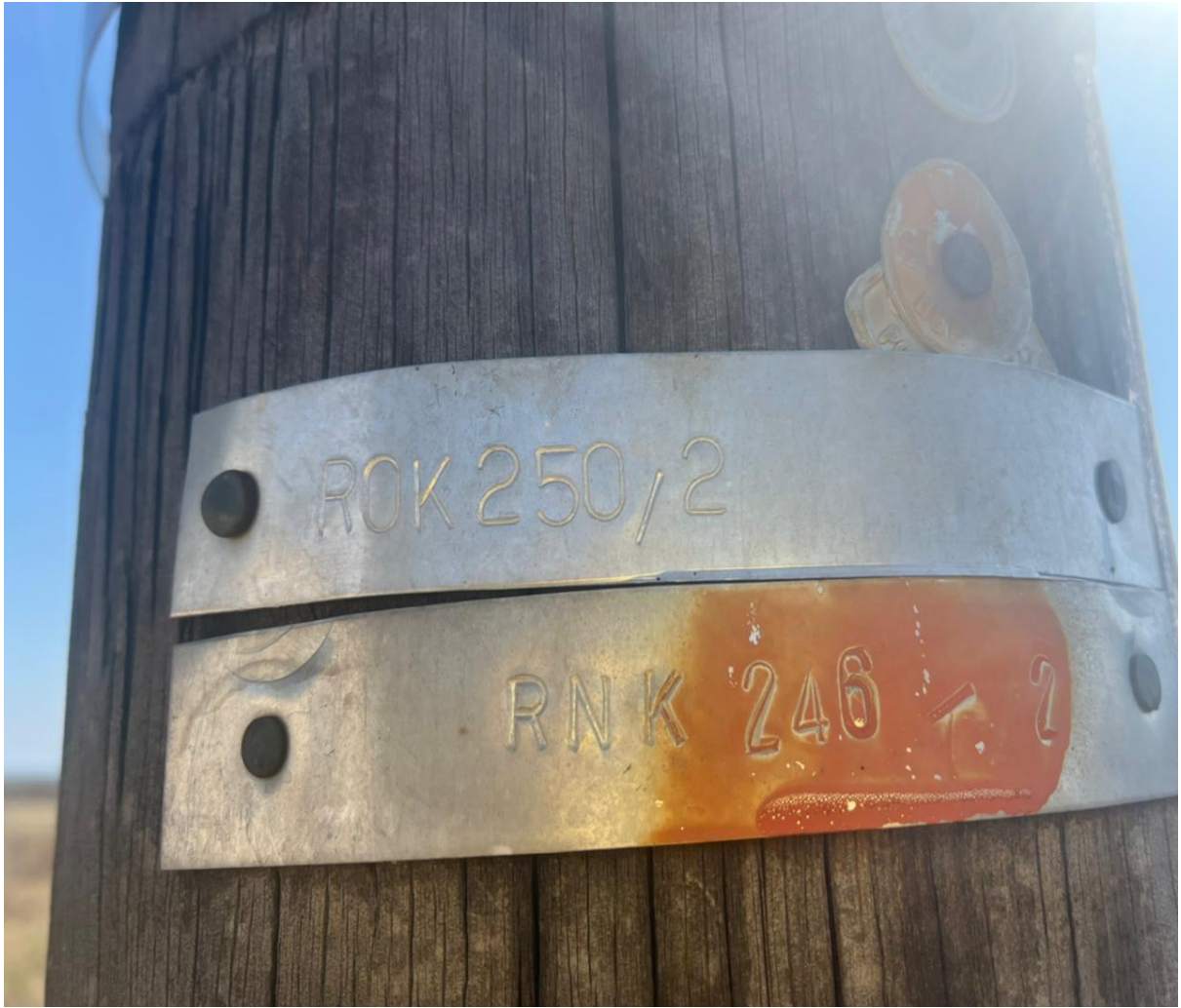
Figure 2: Picture showing pole where the powerline will be supplied from
