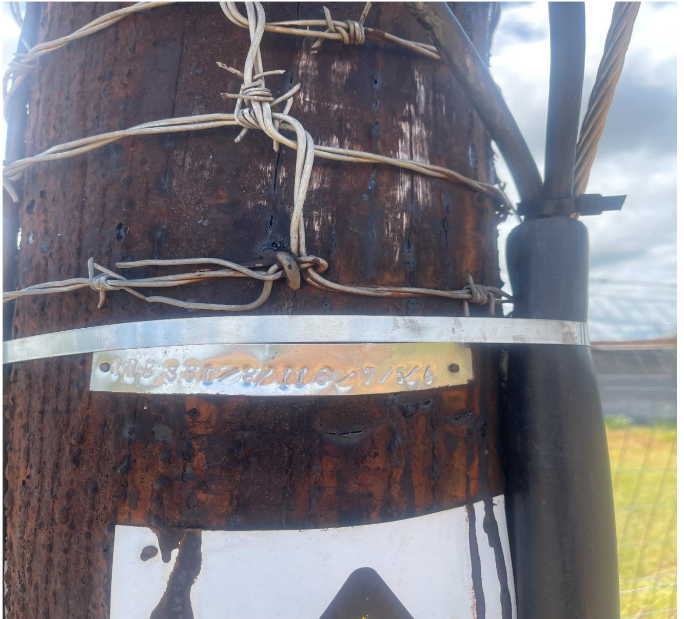
Figure 2: Picture showing existing pole number in the study area
