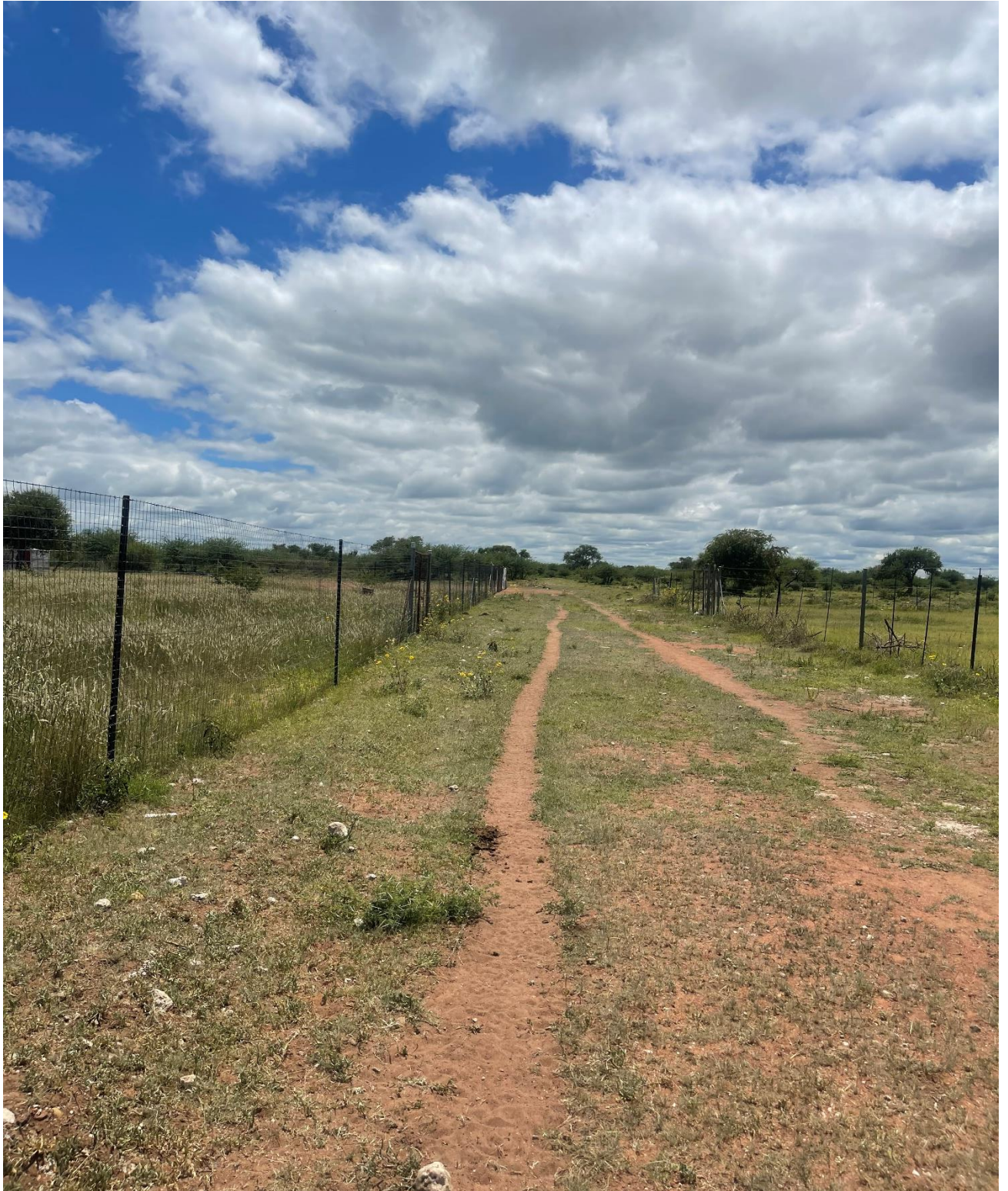
Figure 9: Picture showing road infrastructure in the study area
