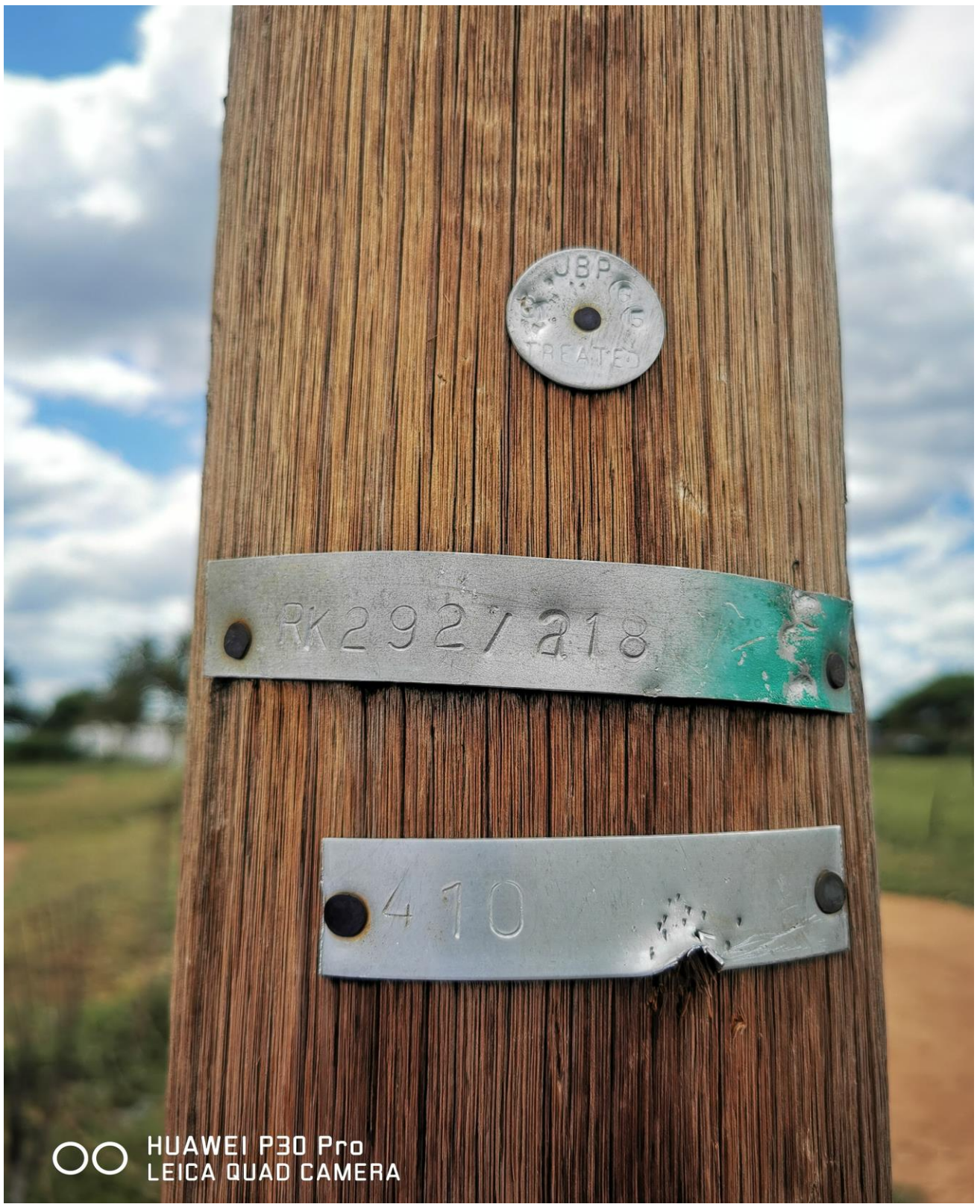
Figure 1: Existing line which the new line will be connected from
