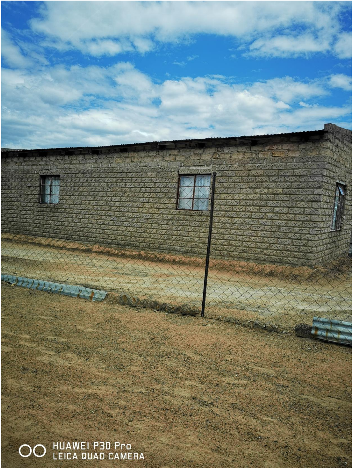
Figure 7: Existing building structure in the project area
