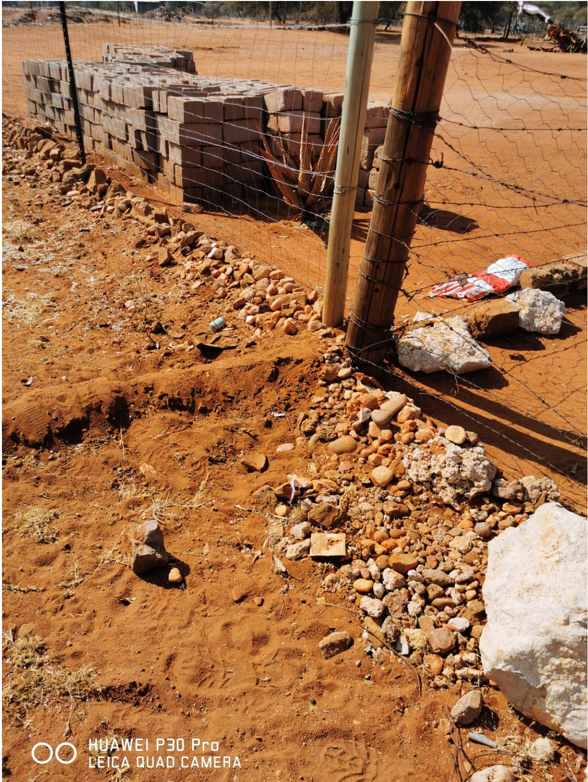
Figure 4: Picture showing one of the line pole position
