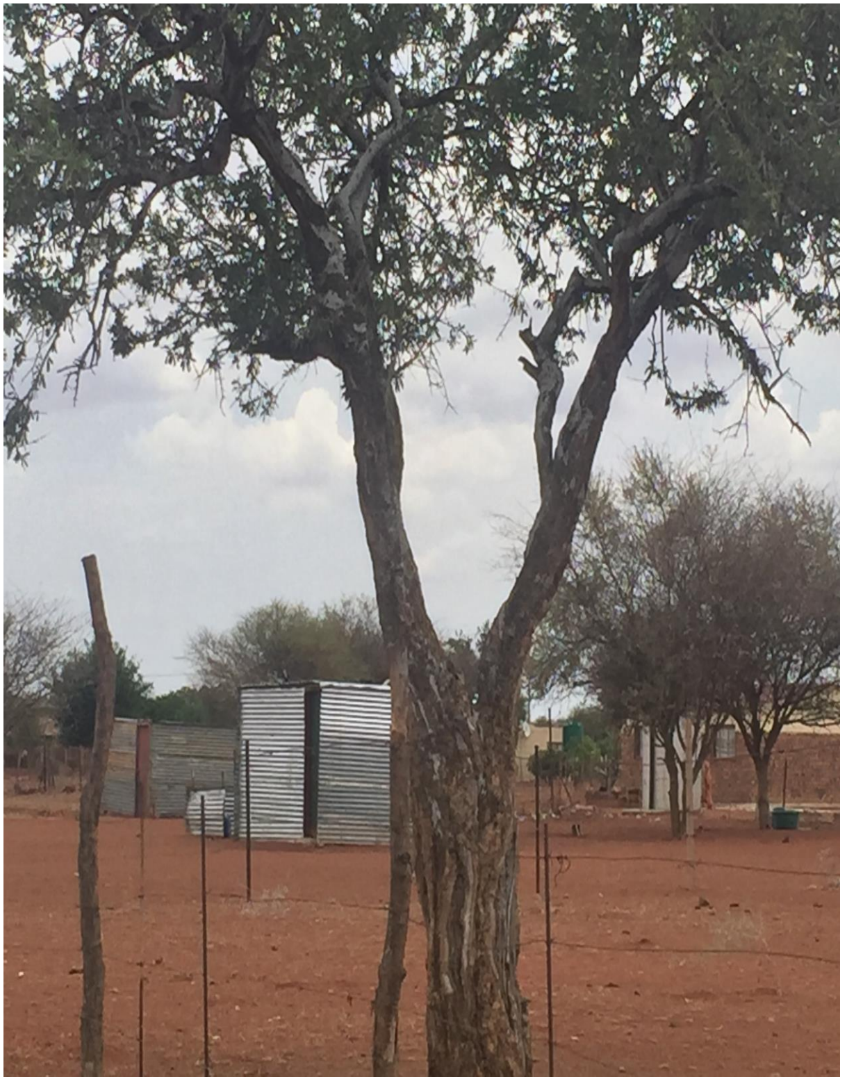
Figure 3: Picture showing the boundary fence and one of the houses to be electrified
