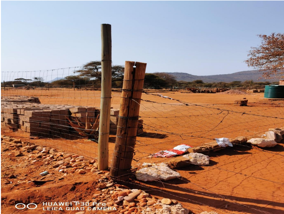
Figure 5: Pegging of LV line
