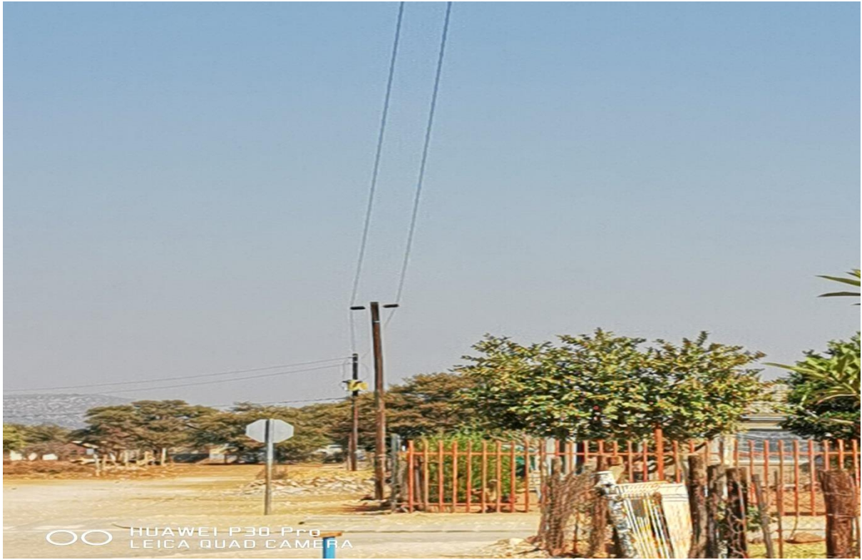
Figure 6: Trees affected and existing powerline
