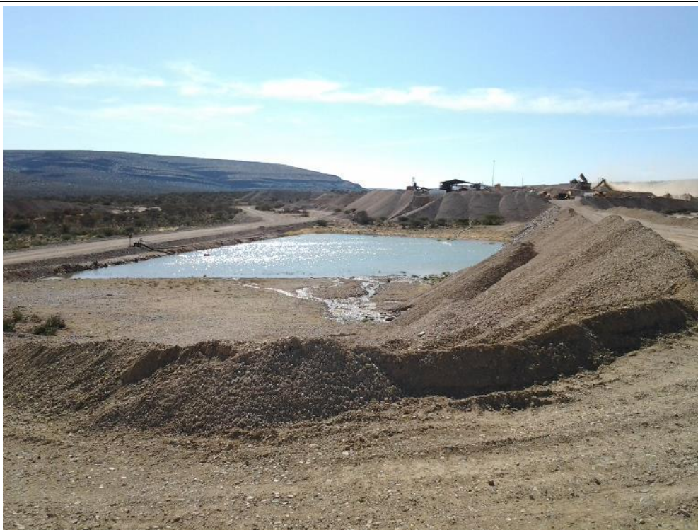
Figure 2: Thunderflex Tailings Storage Facility Return Water Dam.
