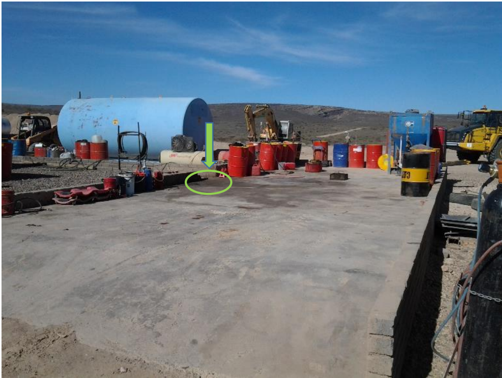
Figure 15: Diamond Recovery Plant equipment wash bay. The location of the silt trap and oil separator is indicated by the green arrow.
