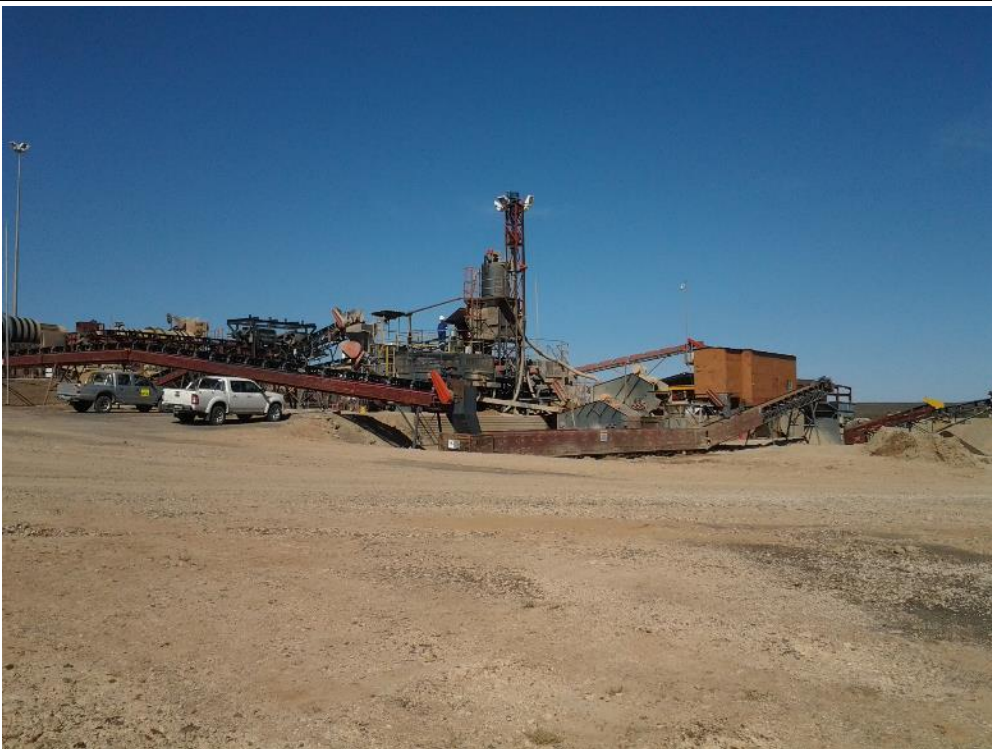
Figure 4: Thunderflex Rotary Pan (RP) Plant viewed towards the south west.
