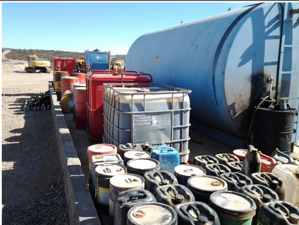
Figure 14: Used oil AST and chemical storage area viewed towards the south west.
