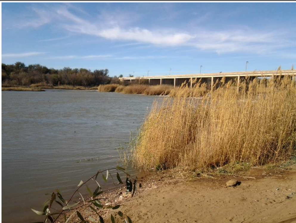
Figure 18: Sample location TSW02 upstream of the Thunderflex operation with the R386 shown in the background.
