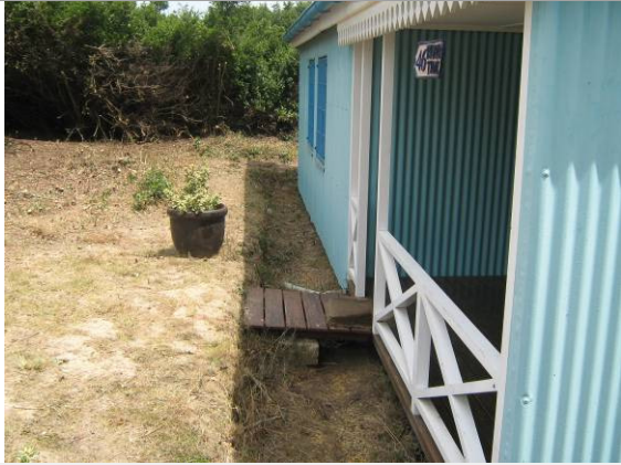
Photo 13: Corrugated iron cottage sunken in, and resting on wooden framework
