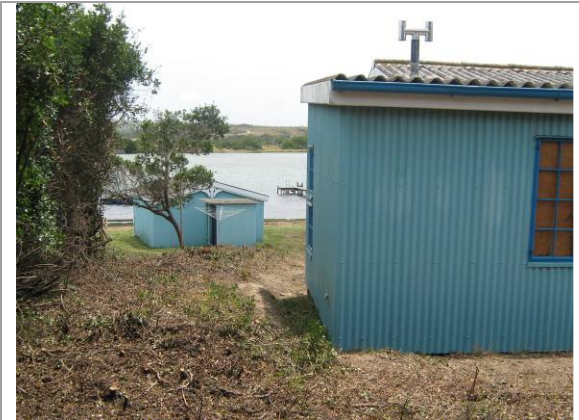
Photo 6: Westerly view towards river, with cleared bush along southern boundary
