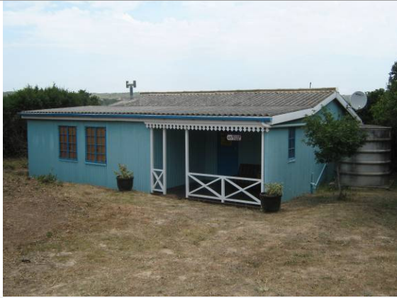
Photo 1: East-facing side of cottage looking towards internal circle road
