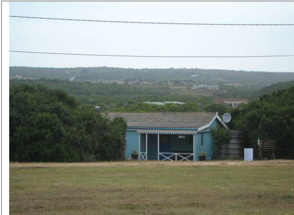
Photo 3: Notice seen from the circular dirt road serving this section of shareblock
