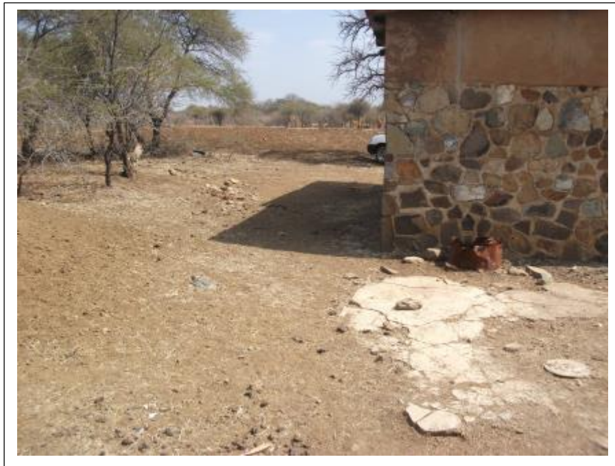
Figure 3- The possible grave may be located next to the piece of cement floor which used to be the floor of the house which Motsabi Alice Pilane occupied. Emily Maretlwa's house is located directly next to the foundation (above).
