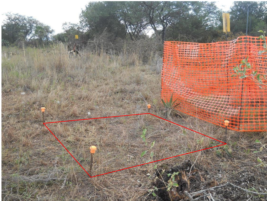
Fig 10. The position of Leg C of Tower 205 is marked with steel rods and yellow caps (indicated with a red square). The burial is temporarily demarcated with the orange netting.
