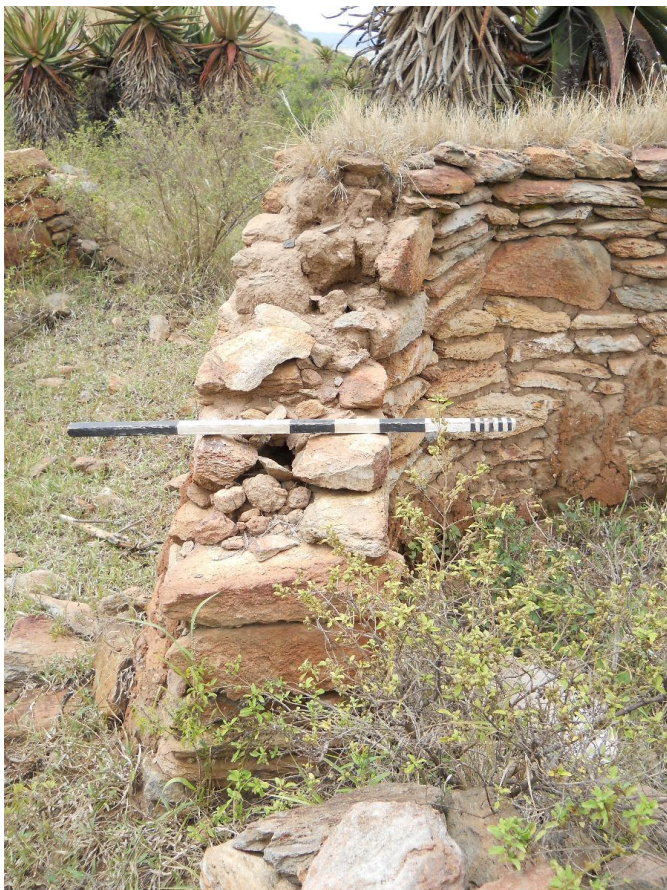
Fig 9. Another characteristic of this later occupation is the mud/clay used in between the stone coursing.
