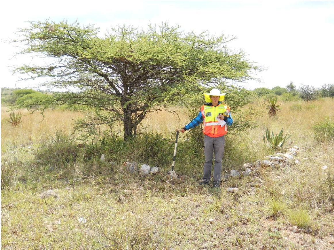
Fig 10. This cylindrical structure ( 23^{\circ}54'11.10''S 29^{\circ}36'47.30''E ) apparently stood on its own. It is mainly built with quartzite. Except for a possible ritual purpose, its function remains speculative unless excavated.
