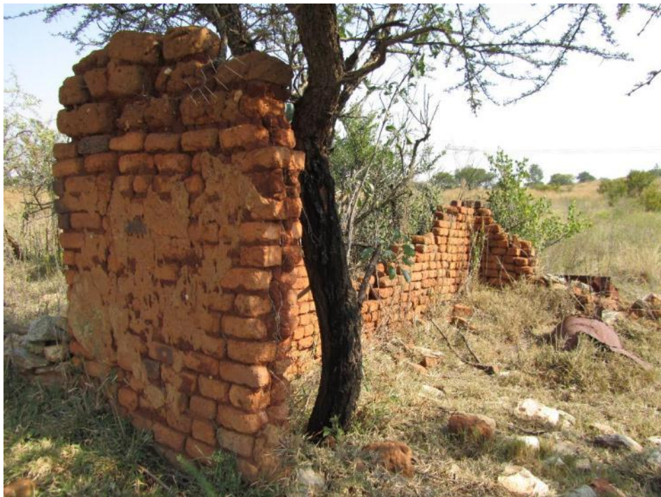
Figure 10. Another rectangular structure built with fired clay bricks. This could probably be younger than the raw brick and stone and dagha structures.
