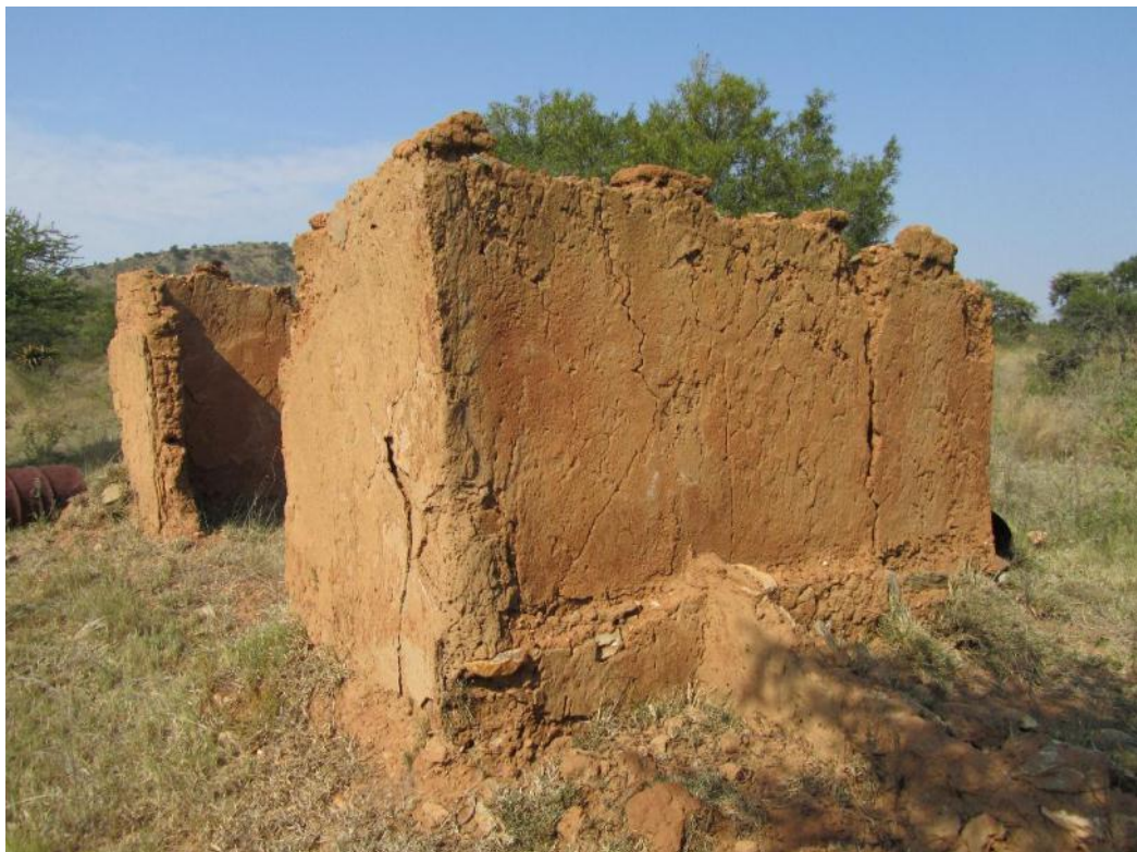
Figure 8. A rectangular structure built with raw clay bricks and plastered with clay. It is possible that this was the first of the rectangular buildings, the later additions built with fired brick.
