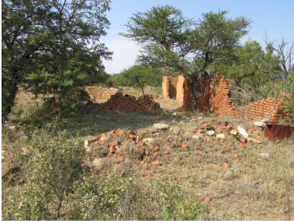
Figure 9. Some of the structures are more recent than the others. This is clearly visible in the stacked clay brick walls, while the walls of the structure in the background have been built with raw bricks and plastered with clay (see Fig 8).
