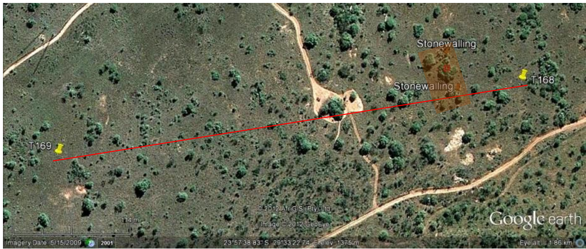
Figure 27. The stone walled structures are in the vicinity of Tower 168, respectively at co-ordinates S23°57'39.0" E29°33'28.2" and S23°57'37.9" E29°33'27.8". It is clear that one of the structures will be impacted on during construction of the line.
