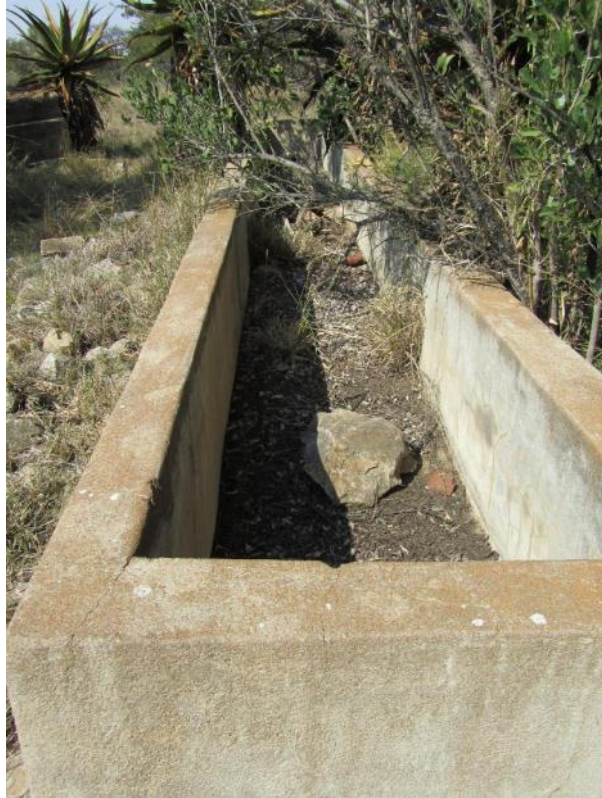
Figure 15. A concrete water trough next to the reservoir.
