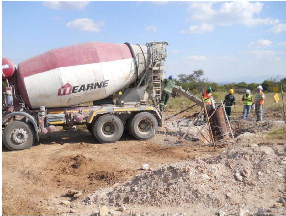
Figure 10. The final stages of the casting process. The archaeologist was also on site, informed about it in advance.
