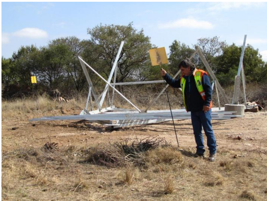
Figure 11. The site on May 22: Mr O De Canha is standing at the site of the one grave with one of the yellow markers in his hand. This was picked up in the veldt beyond the construction material. No demarcation is in place and it is evident that vehicles were driven over it.
