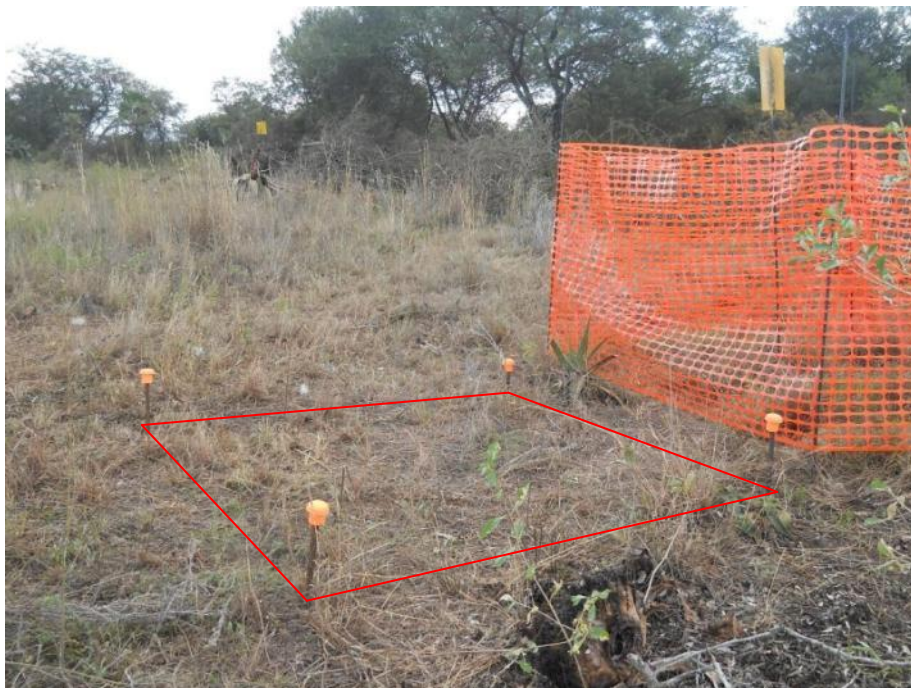
Figure 3. The position of Leg C of Tower 205 is marked with steel rods and yellow caps (indicated with a red square). The burial is temporarily demarcated with the orange netting. From the above image it is clear that the one leg of the tower is almost on top of the grave.
