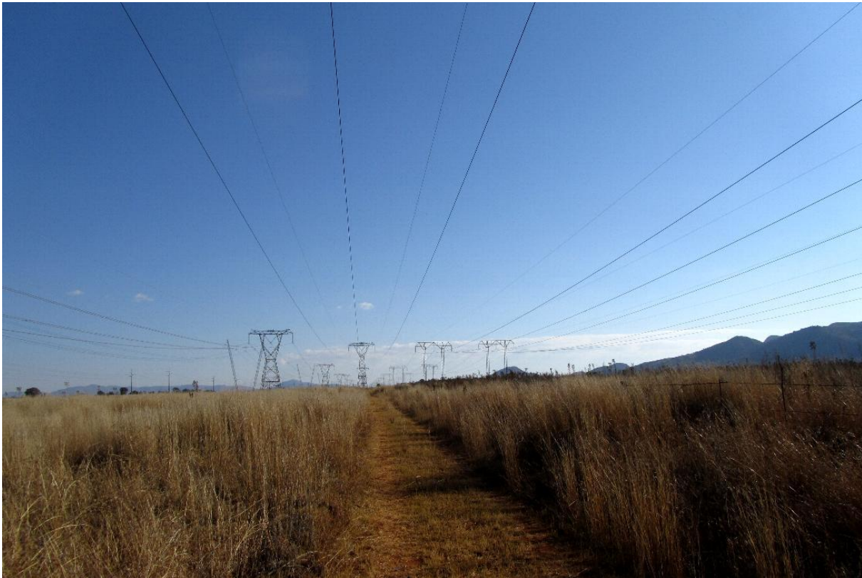
Figure 15. The relatively wide area covered by several power lines. It is clear that these lines impact upon large areas of the landscape, whether it is natural or human-made. It is thus obvious that laws pertaining to the protection and preservation of archaeological sites are not excessive or unnecessary.
