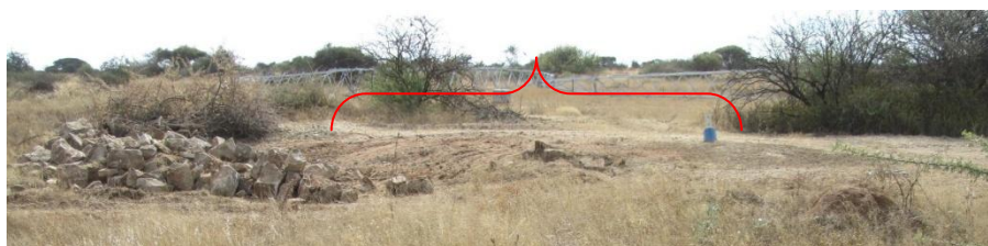
Figure 2. Only a small part of the dam was compromised when the stacked rocks were moved a few metres. The original position is indicated with the brace.
