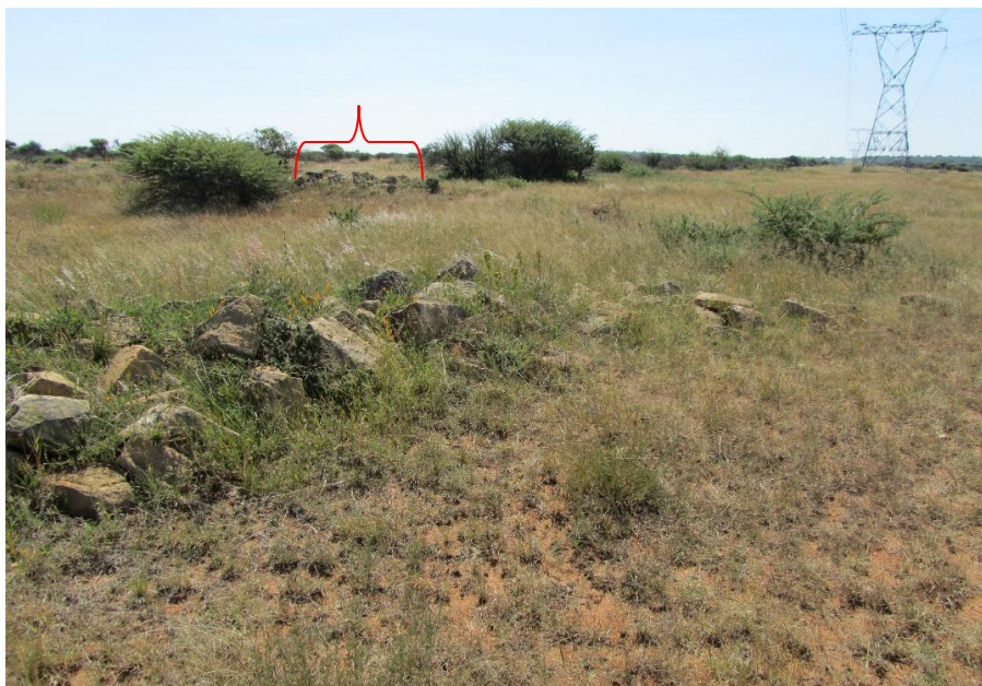
Figure 1. The stone-walled farm dam. The retaining wall consisted of roughly stacked rock. Only a small area (indicated by the brace) was moved to make place for the foundation of the tower's one leg.
