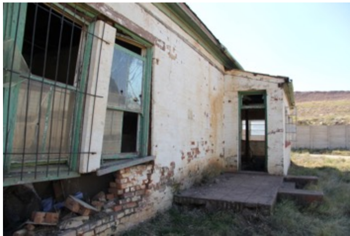
Figure 8: Front end of the original Office Building at Simmer and Jack.
