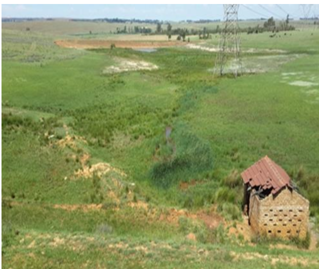
Photo # 5 : Smaller dam downstream the main dam
