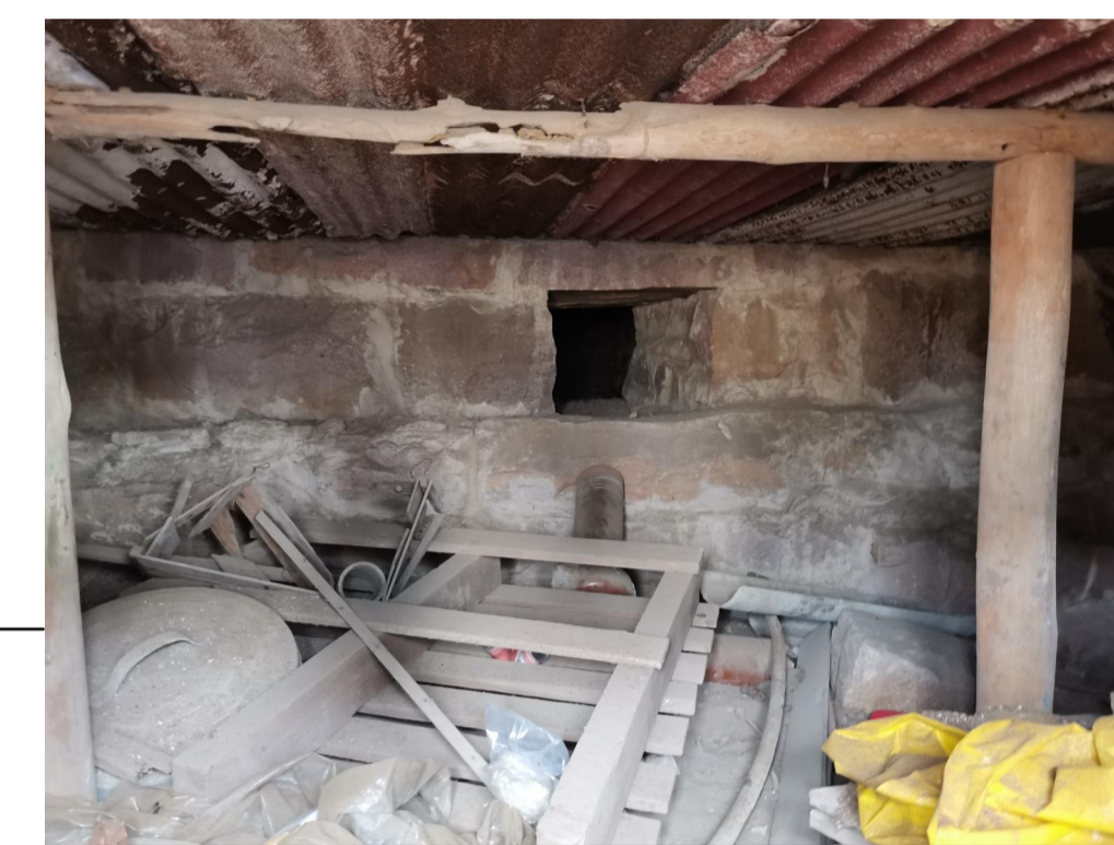
EXISTING SOUTHERN VENTILATION HOLE IN EXISTING STONE WALL
