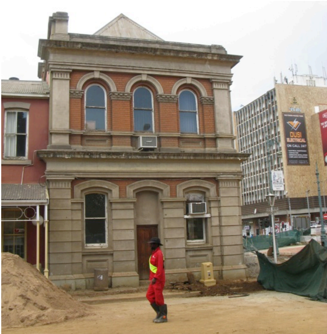
Part north-west corner of Publicity House facing City Hall
