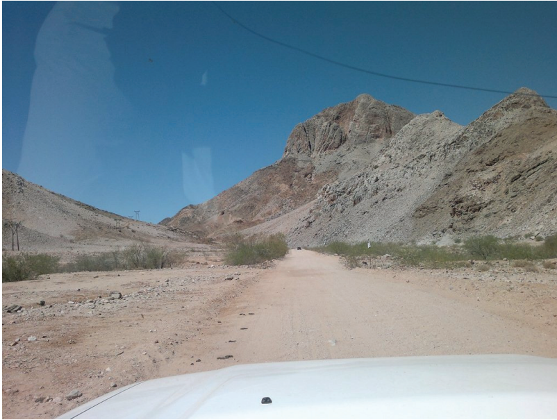
Pipeline exit riverbed area to pump station
