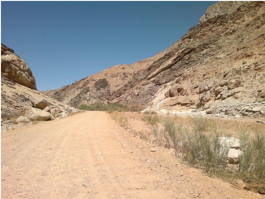
Pipeline in riverbed area - pipeline on right
