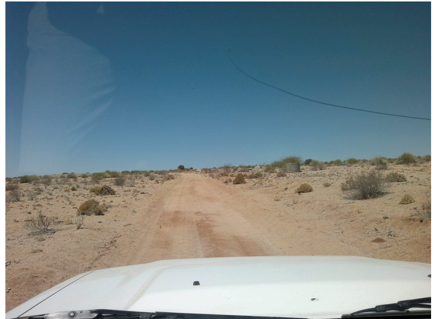
Pipeline on Right hand side (chamber valve)
