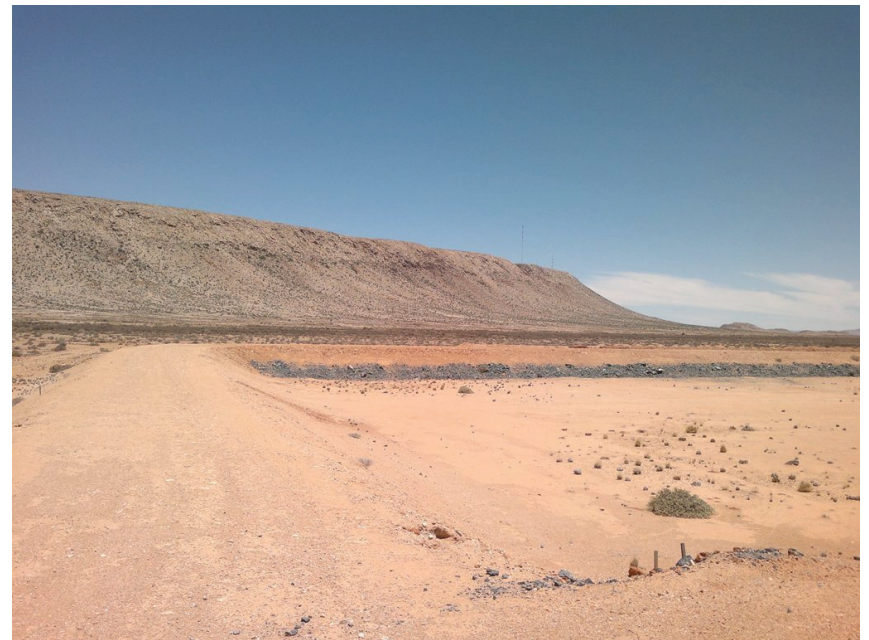
Gamsberg evaporation pond – possible location for reservoir 2
