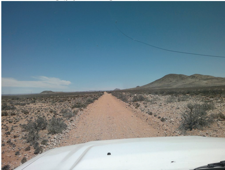
Servitude with pipeline on right
