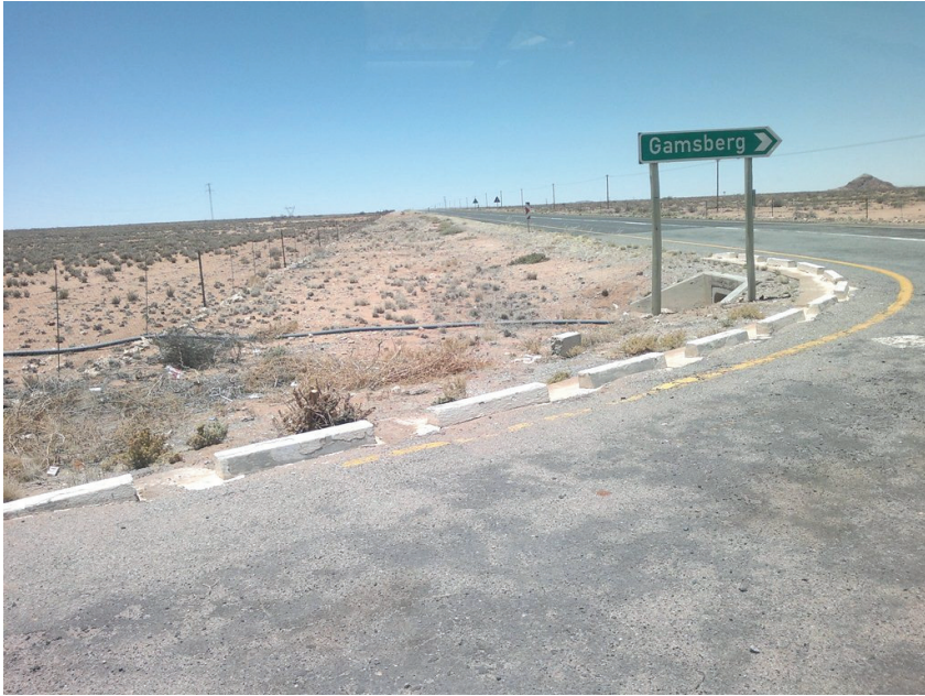
Pipeline N14 Crossing
