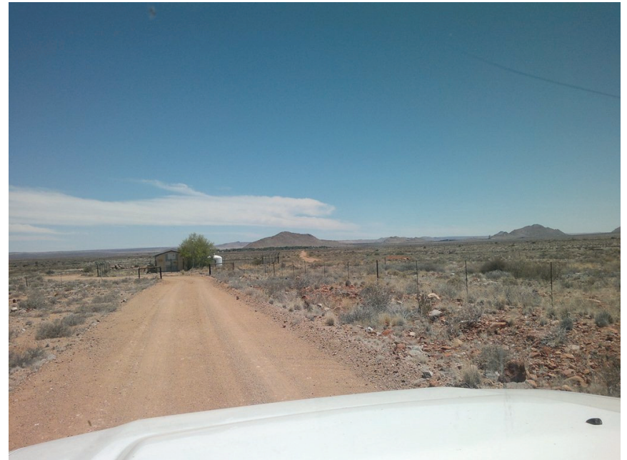
Servitude, road and kokerboom pump station
