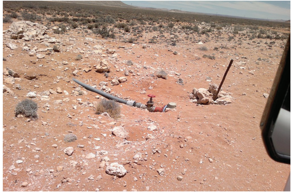
Existing small take-off for new pipeline installation
