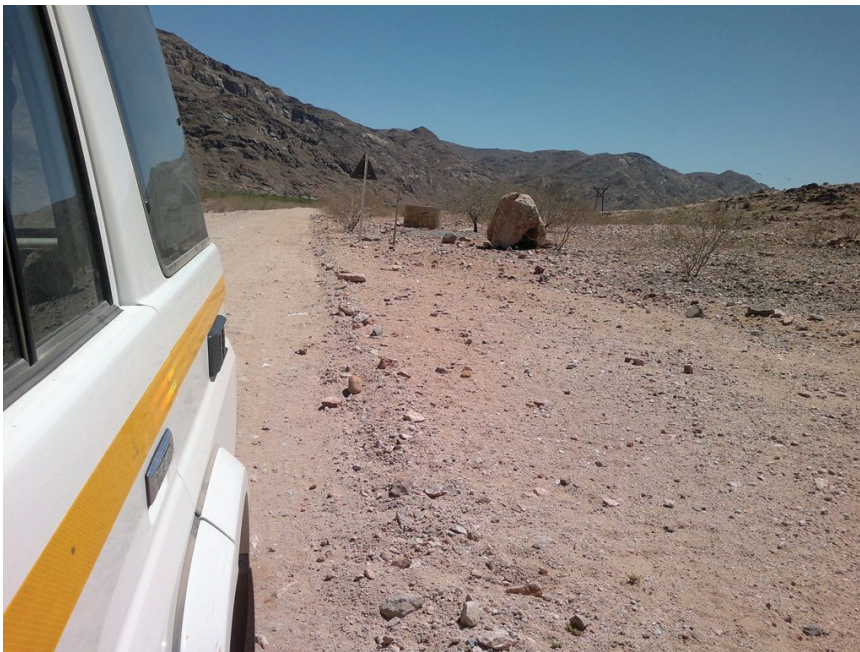
Pipeline crossing over under road (left to right)
