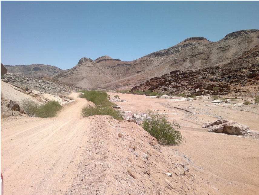
Pipeline in riverbed area - pipeline on right
