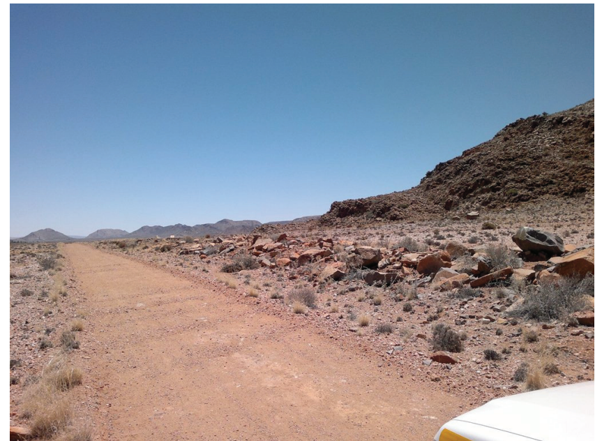
Servitude Road with blasted material on road verge
