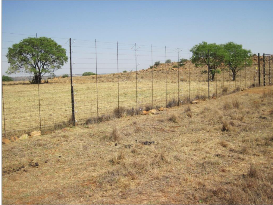
Figure 5: The sturdy game fence marking the southern border of the to-be-affected property (Zwavelpoort 373 JR, the Brown demarcated property, Figure 1) consisting of ample droppers, barbed wire, horizontal steel strands, a wire mesh and the isolated electrical wires.
