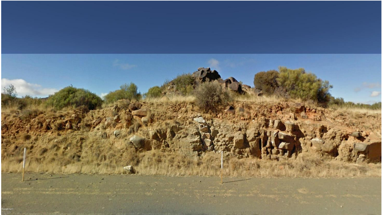
Figure 9 Dolerite weathering profile with corestones and surface boulders (N10 near the Mooi Plaats site – Google Earth)
