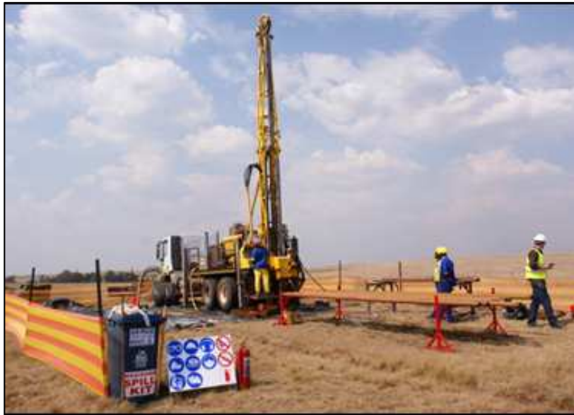
Figure 3: Typical Drill Site
