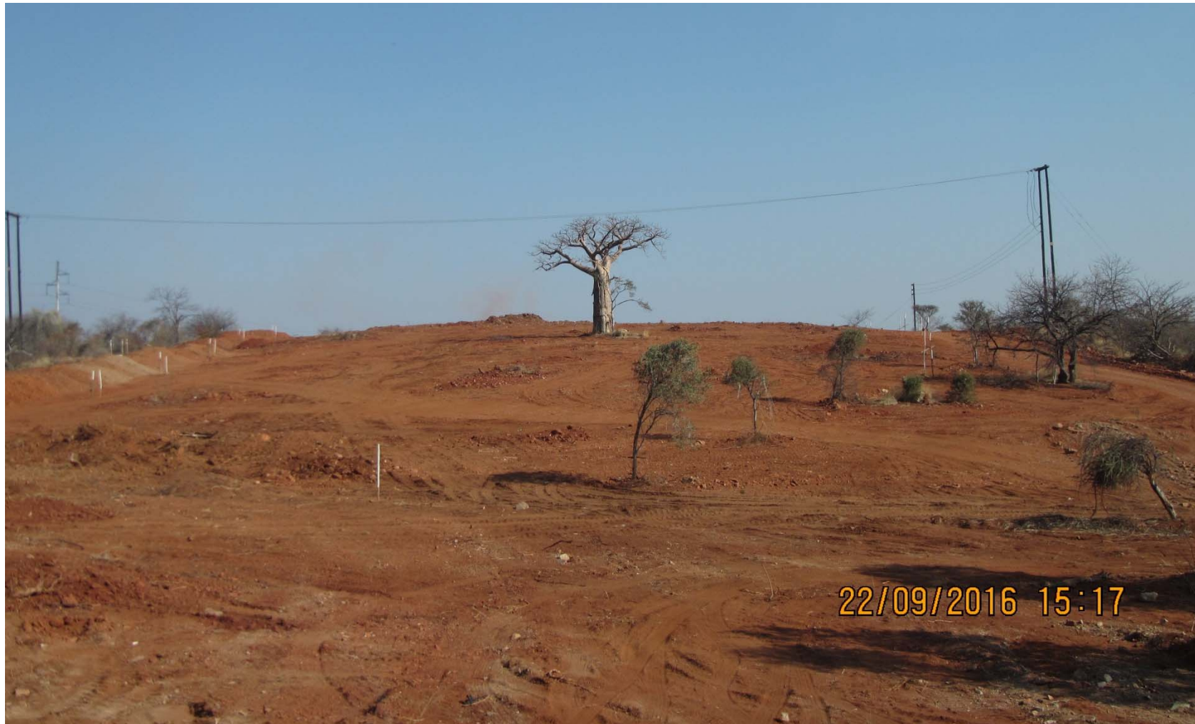
Figure 4-24: N1 by-pass under construction
