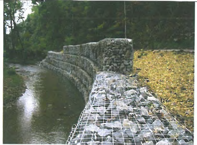
Gabion baskets can be used to stabilise banks
