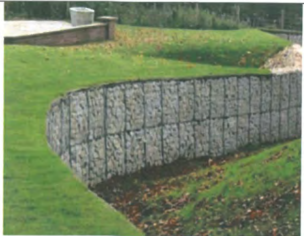
Box gabions can be used to stabilise river banks
