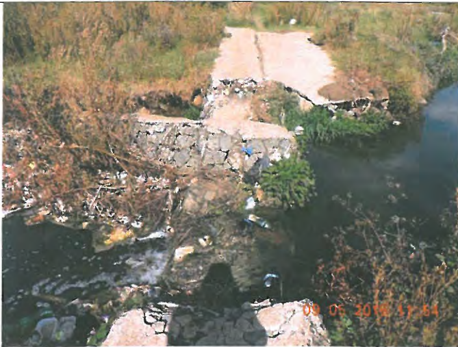
Gabion collapse at the Jabavu section
