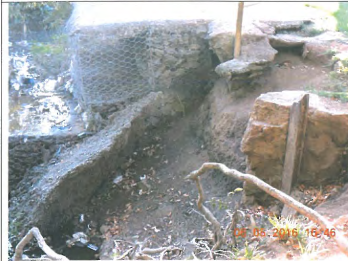
Collapsed gabions
