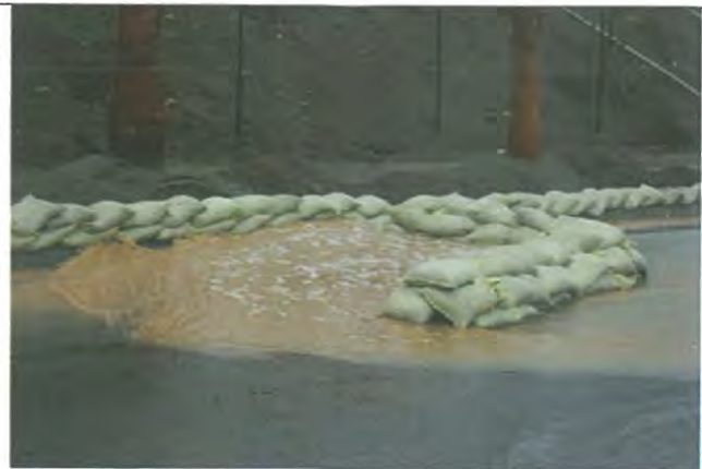
Use of gravel bags to combat sedimentation
