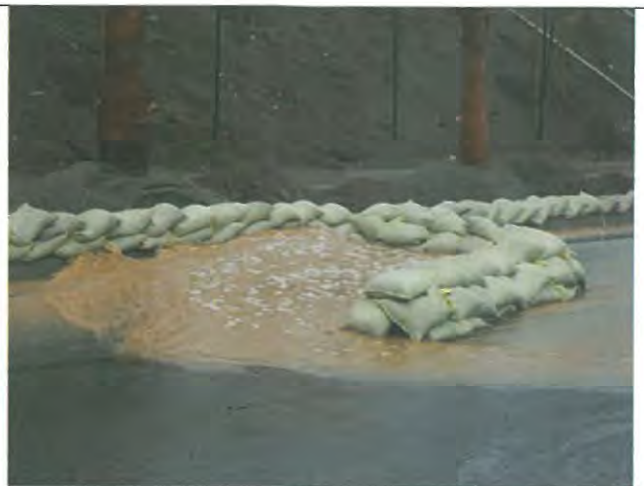
Use of gravel bags to combat sedimentation
